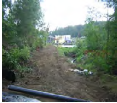
Creek Channel Before
