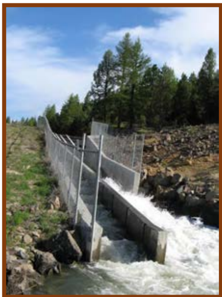
Photo 3. Bates Pond fish ladder. Courtesy of ODFW.
