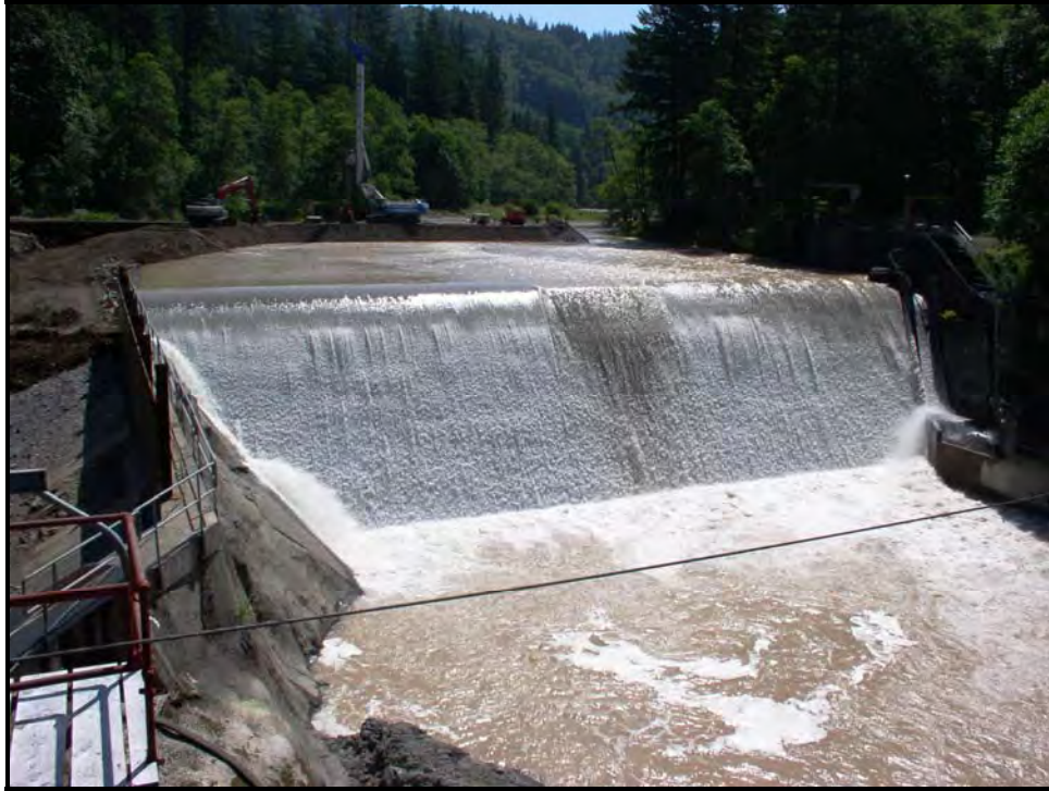
Figure 1-2. Marmot Dam full to the top with sediment, prior to removal, summer 2007.
