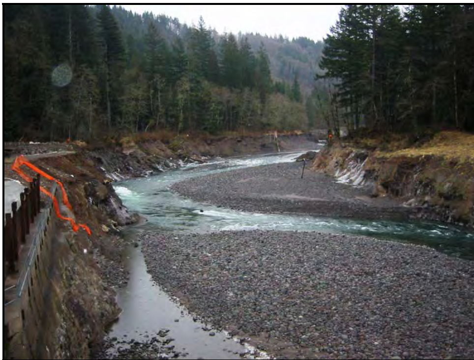
Figure 1-3. Former Marmot Dam site as it appeared in January 2008.
