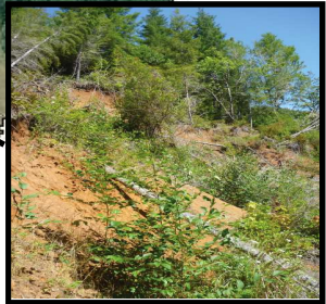
Landslide that occurred in the Upper Wood Treatment reach during winter 2006 / 2007.
