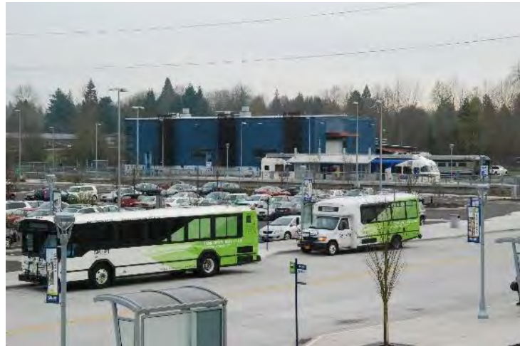
Figure 2-8. SMART Transit Center, Wilsonville
