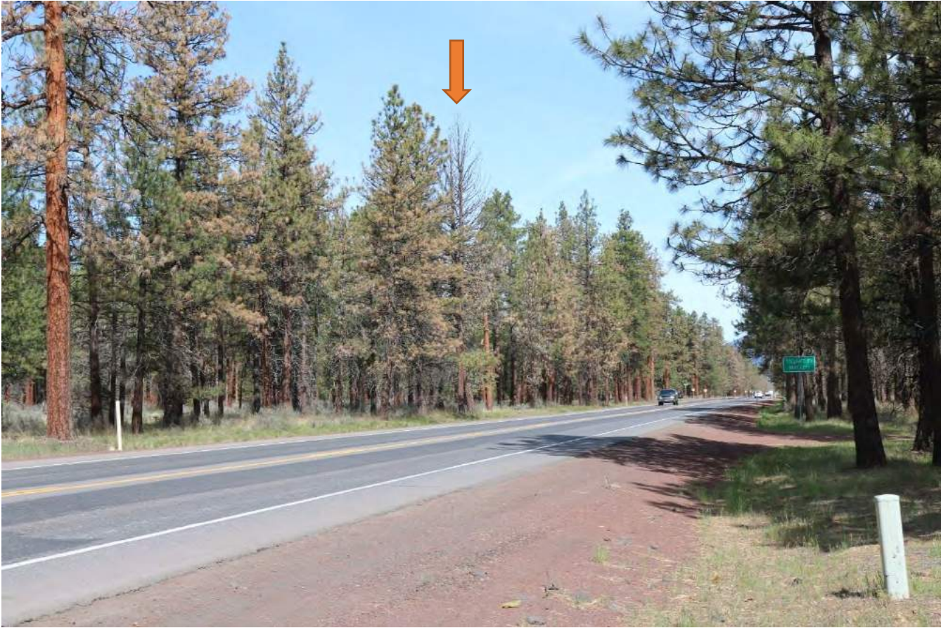
Figure 1b. Increased damage in ponderosa pine along Highway 20 three years later– taken at the same location as the photo in Figure 1a on May 3, 2018. Arrow for reference in Figure 1a.
