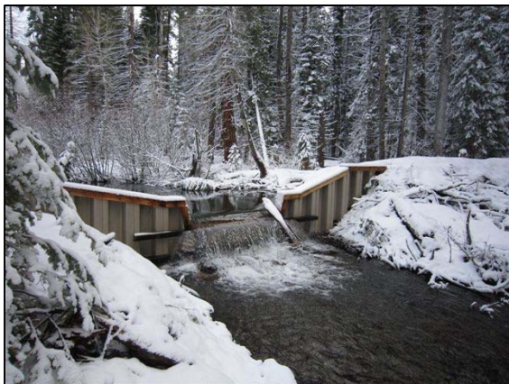
One of two barriers constructed on Sun Pass State Forest during 2010 and 2011 to exclude non-native fish (photo: Dave Hering).
