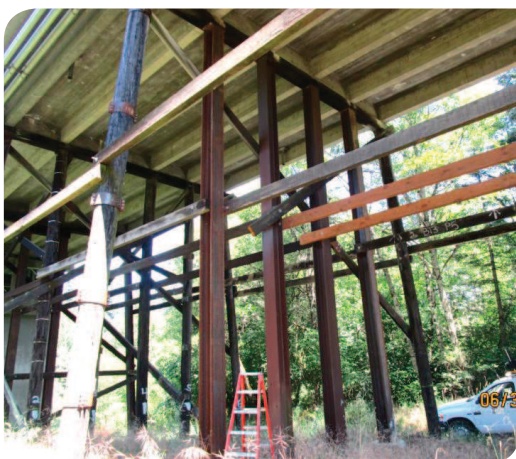
Repaired timber pile at South Yamhill River Bridge.
