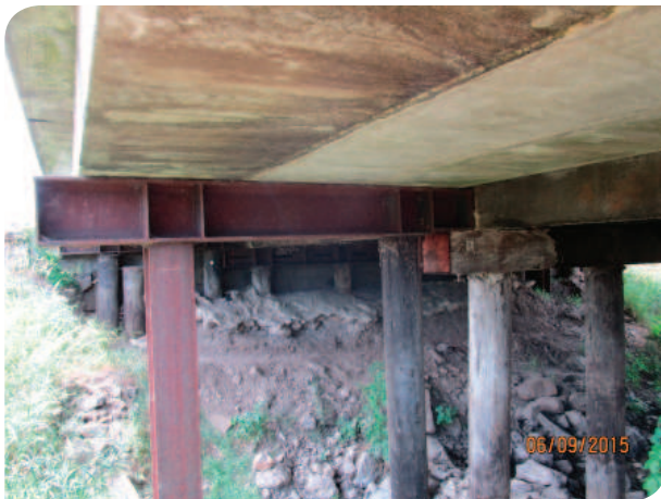
Repaired timber pile at Flat Creek Bridge.
