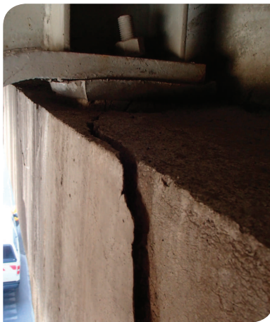
Damaged bridge bearing ledge.
