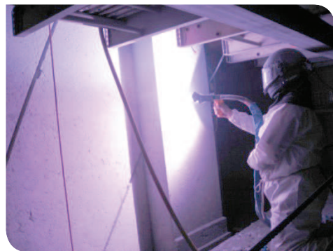
Cathodic protection application (zinc).
