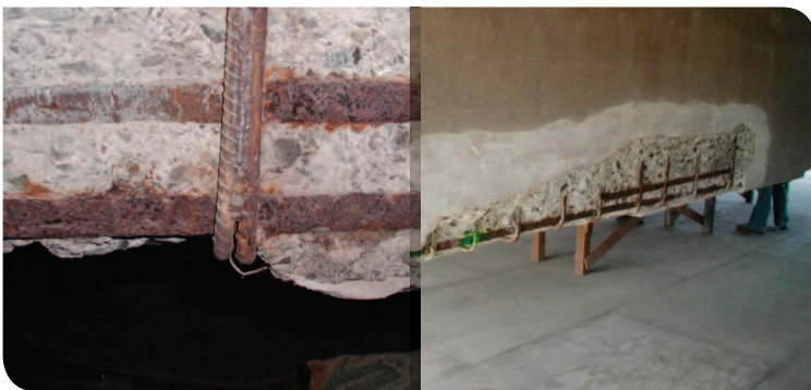
Corroded reinforcing steel prepared for cathodic protection.
