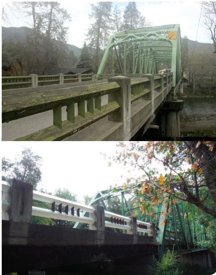
Rail Repair: Applegate Pioneer Bridge
