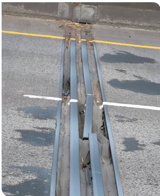
Damaged bridge joint
