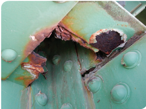
Corrosion damage on Old Youngs Bay Bridge
