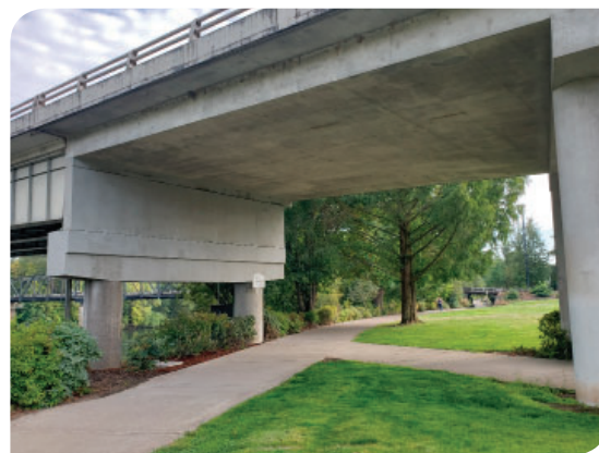
Repair complete. The poor concrete has been patched and the wall sealed to keep water from reaching the reinforcement.
