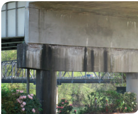
Water seeping through support wall from the open joint above.
