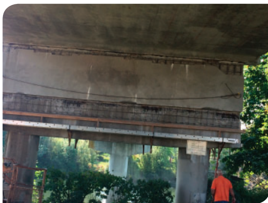
The support wall and crossbeam are prepared for patching. Poor concrete is saw cut and removed leaving neat lines for the new patching material.
