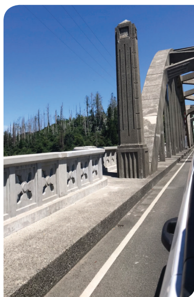
Retrofitted bridge rail.
