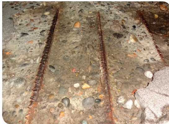
Spalled deck concrete.
