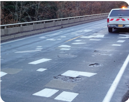
Thin overlay failing due to corrosion.
