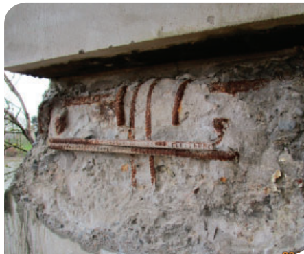
Close up of crossbeam under the support wall. Concrete is spalling leaving exposed reinforcement.
