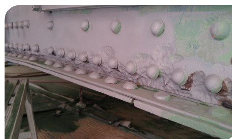
Failed paint on steel member.
