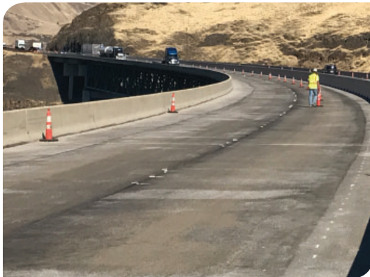
John Day River Bridge deck overlay preparation.
