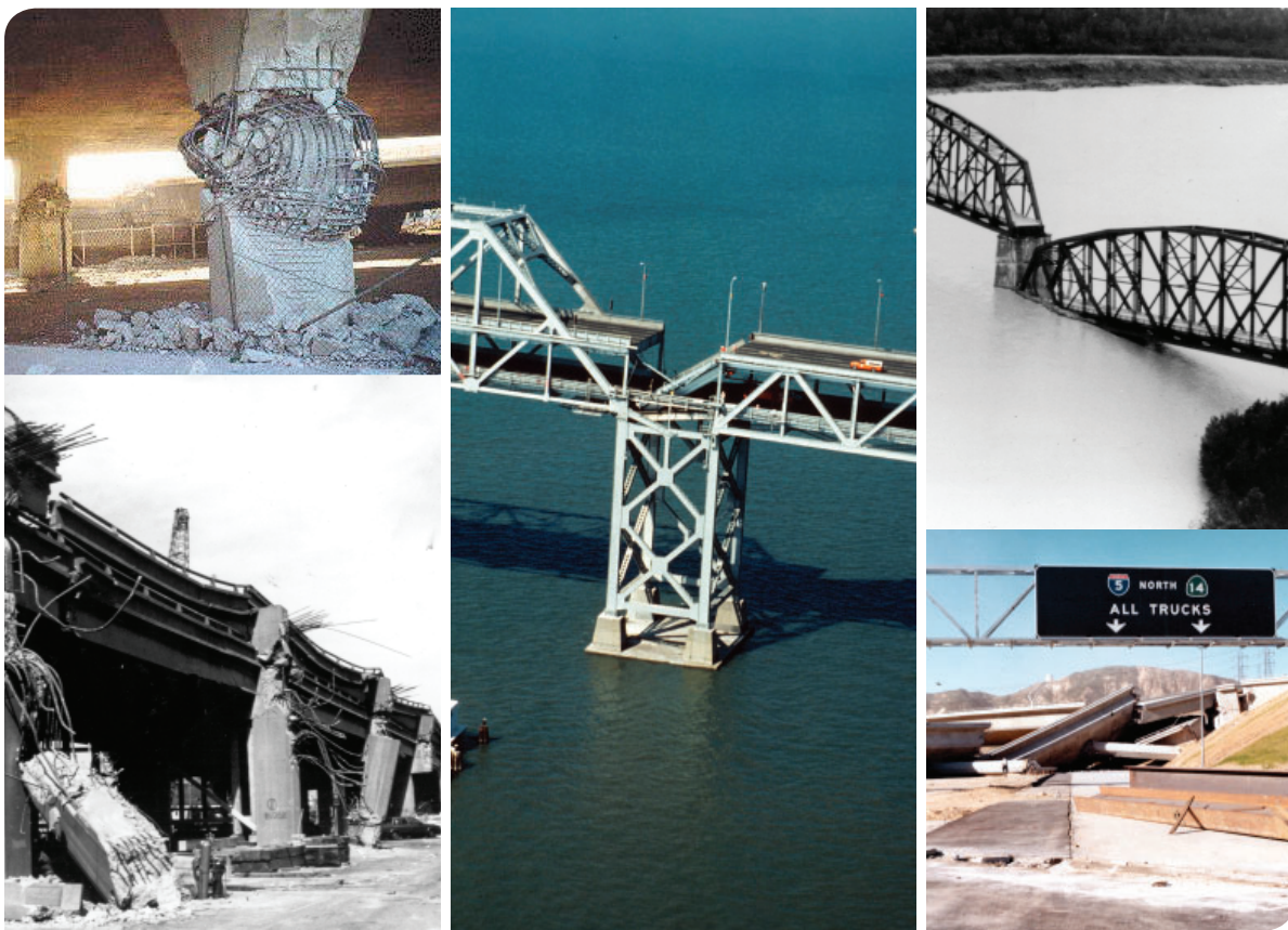
Bridge damage caused by historic earthquakes. Photos courtesy of USGS.
