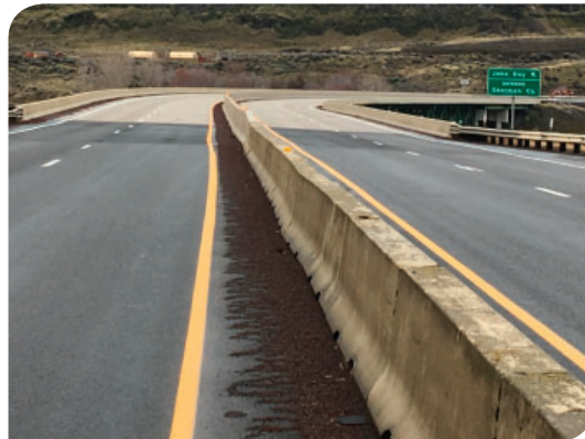
John Day River Bridge deck overlay completed.
