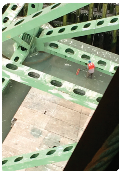
Painting preparation on the Astoria Megler Bridge.
