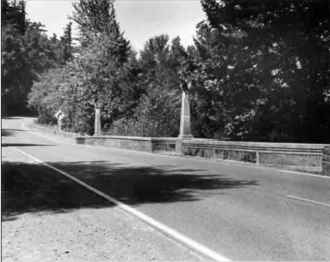
Structure Number 11113 Constructed – 1915 Stark Street Reinforced Concrete Deck Arch Gresham vicinity, Multnomah County Ownership – Multnomah County
