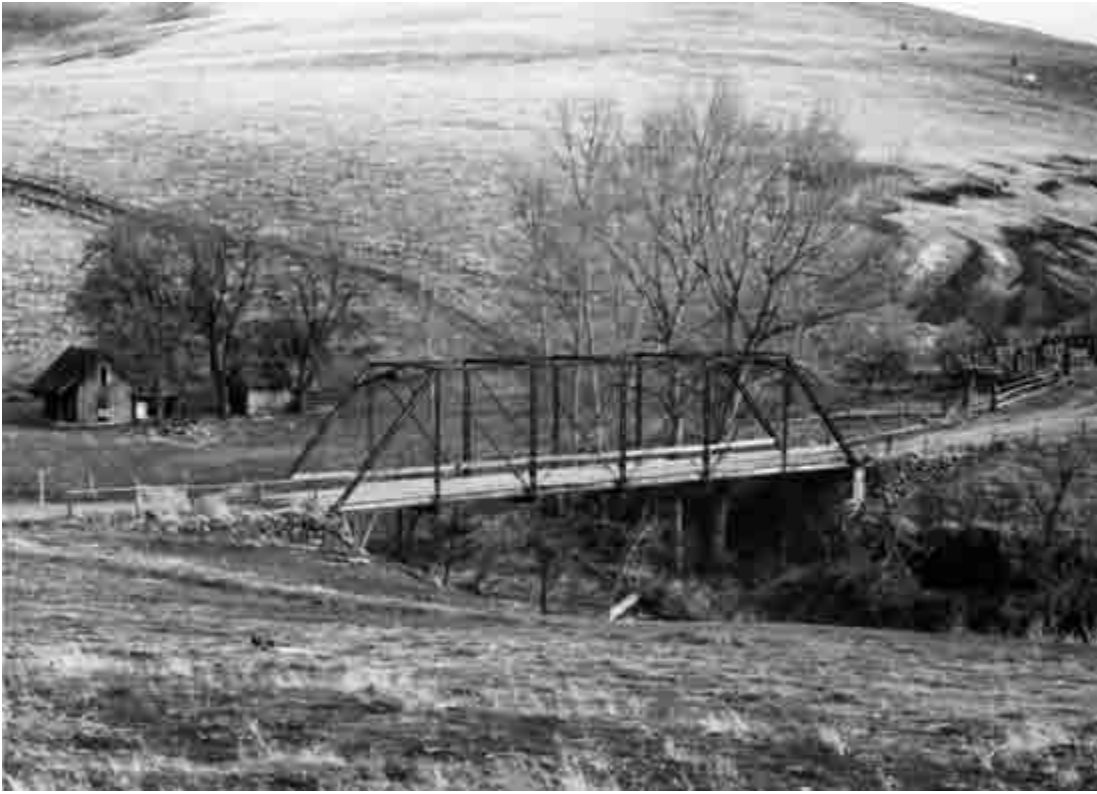
FIGURE 19. Bridges relate aesthetically to the landscape. The pastoral setting of the Rhea Creek Bridge (1909) near Ruggs in Morrow County increases its appeal and significance.
