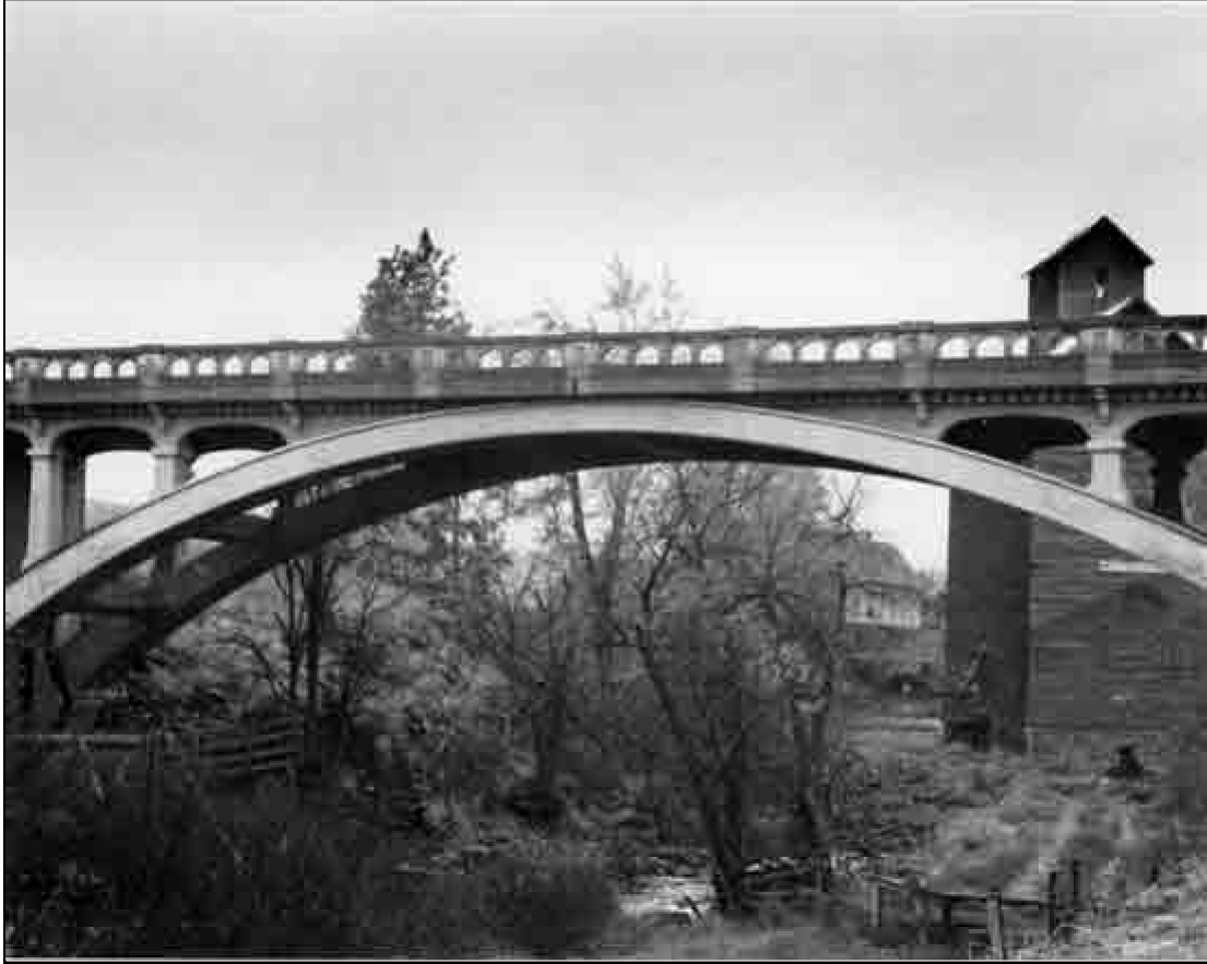
Structure Number 1095 Constructed – 1925 Boyd County Road Reinforced Concrete Deck Arch Boyd vicinity, Wasco County Ownership – Wasco County
