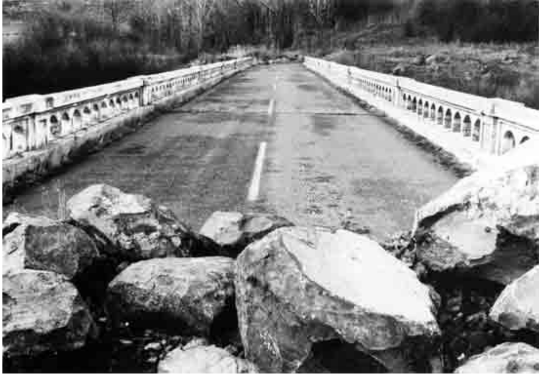
FIGURE 25. The Old Rhinehart Bridge (1922) across the Grande Ronde River in Union County is bypassed and abandoned-in-place, one of many methods for preserving historic bridges in Oregon.
