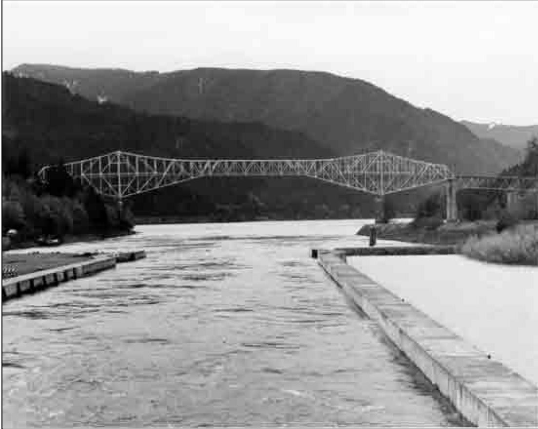
Structure Number 02592 Constructed – 1926 Bridge of the Gods Road Steel Through Truss (Cantilever) Cascade Locks, Hood River County (Oregon) and Ownership – Port of Cascade Locks Stevenson vicinity, Skamania County (Washington)
