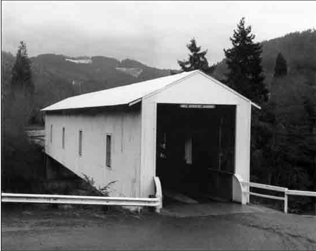
Structure Unnumbered Constructed – 1962 Milo Academy Private Road Steel Through Girder Covered Bridge Days Creek vicinity, Douglas County Ownership –Private
