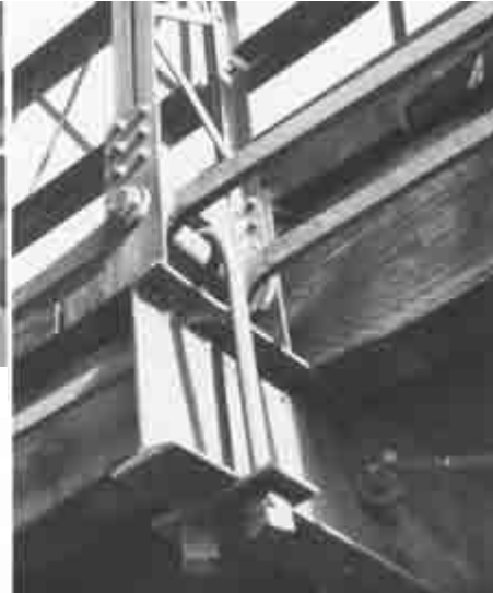
Pin connection on a steel truss (detail).
