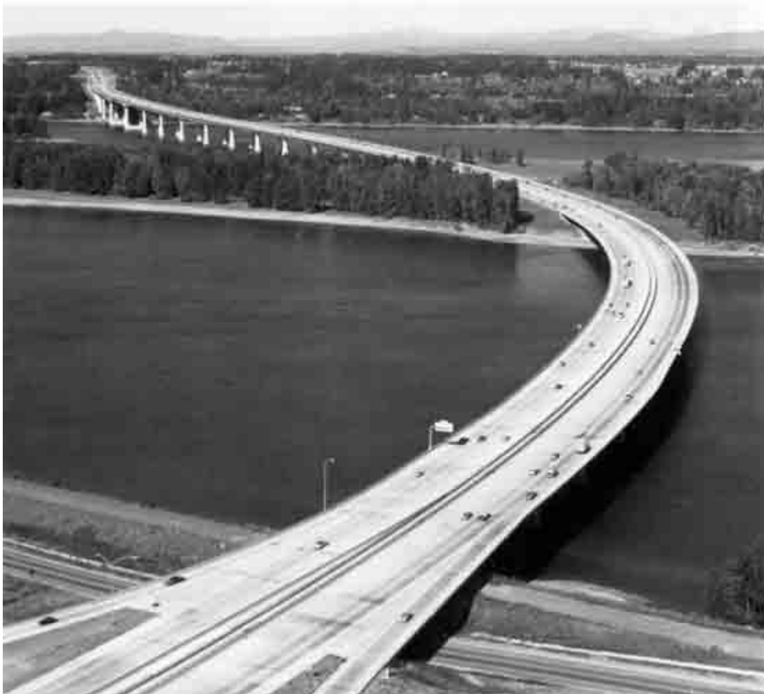
FIGURE 14. Oregon's latest spectacular addition to its bridge-building tradition is the Interstate 205 crossing of the Columbia River, completed in 1982. Dedicated to Glenn L. Jackson, long-time member of the Oregon Transportation Commission, the twin structures are post-tensioned reinforced concrete box girders, 11,750 feet in length.
