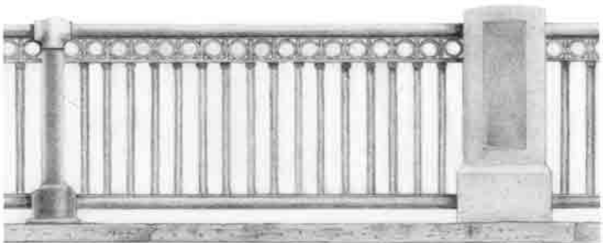
St. John's Bridge (1931), Willamette River, Portland, Multnomah County
