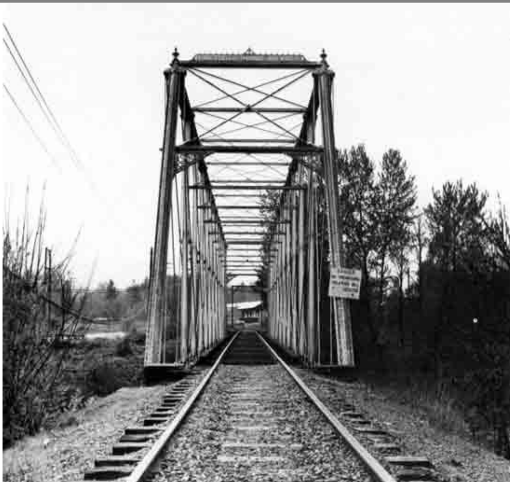
FIGURE 10. The Booth-Kelly Railroad Bridge (also called the Hayden Bridge) across the McKenzie River at Springfield is considered the oldest surviving bridge in Oregon. The wrought iron truss structure was first erected near Corrine, Utah, in 1882 and was moved to its present location in 1900. The Whipple truss and Phoenix columns make it a unique structure. It is now a public footbridge.
