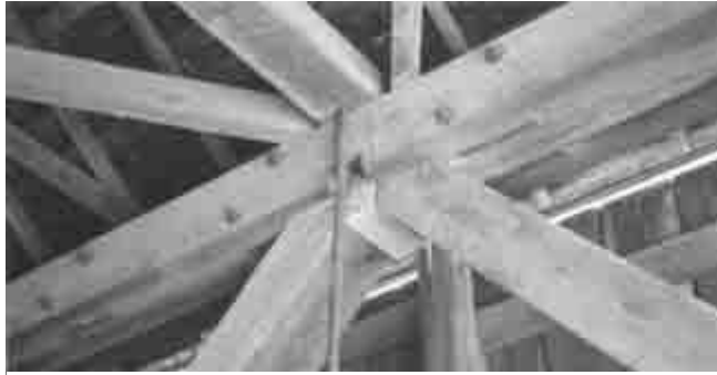
Timber truss joint on a covered bridge (detail)
