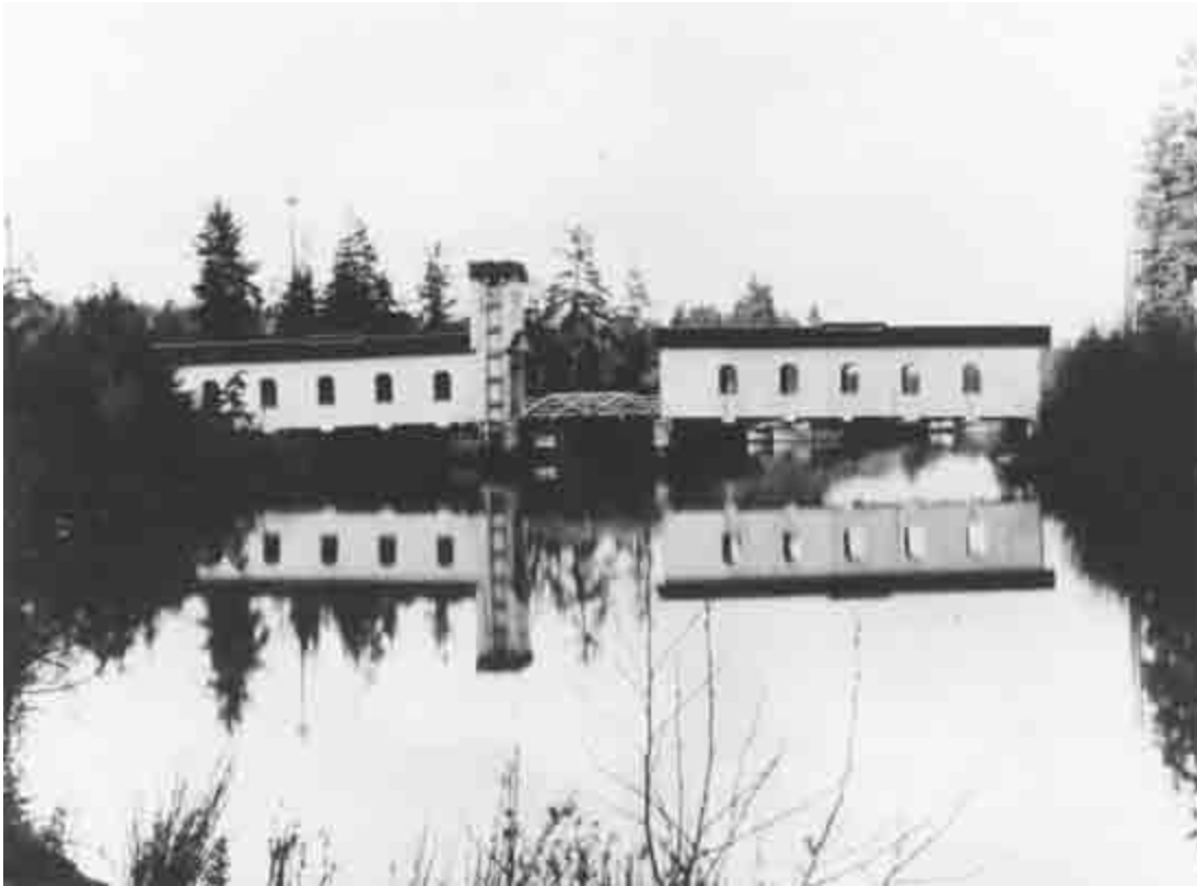
FIGURE 6. An early small bascule bridge in Oregon was the John Day River Bridge, constructed on the Lower Columbia River Highway near Astoria, Clatsop County, in 1918. The timber truss bascule opening span was flanked by two timber truss covered spans.
