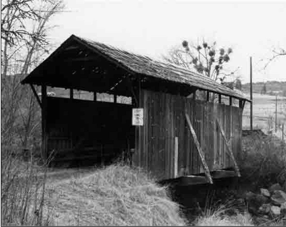
Structure Number 29C262 Constructed – 1919 Lost Creek County Road Timber Through Truss (Queenpost) Lakecreek vicinity, Jackson County Ownership – Private
