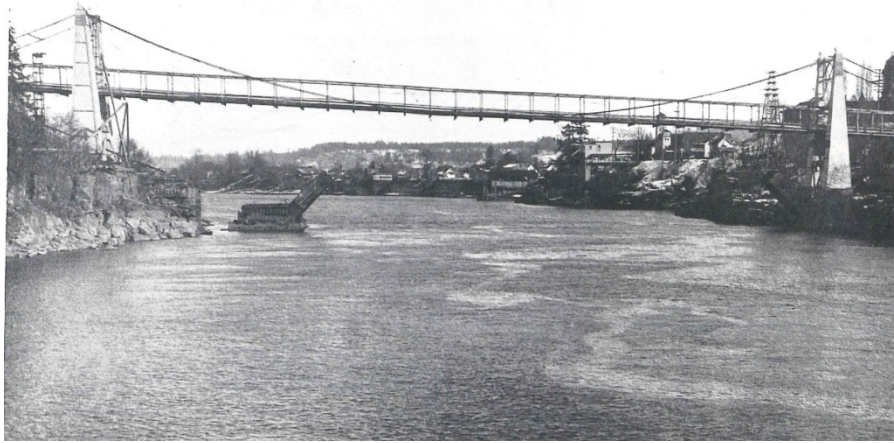
FIGURE 5. A suspension bridge across the Willamette River was built in 1888 at Oregon City. One of only a few large suspension bridges in Oregon's bridge-building history, the narrow bridge was replaced in 1922 by a steel arch span.
