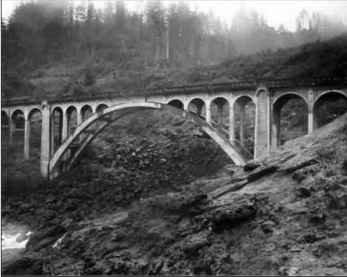
Structure Number 1089 Constructed – 1927 Otter Creek Loop Road Reinforced Concrete Deck Arch Otter Crest vicinity, Lincoln County Ownership – Lincoln County
