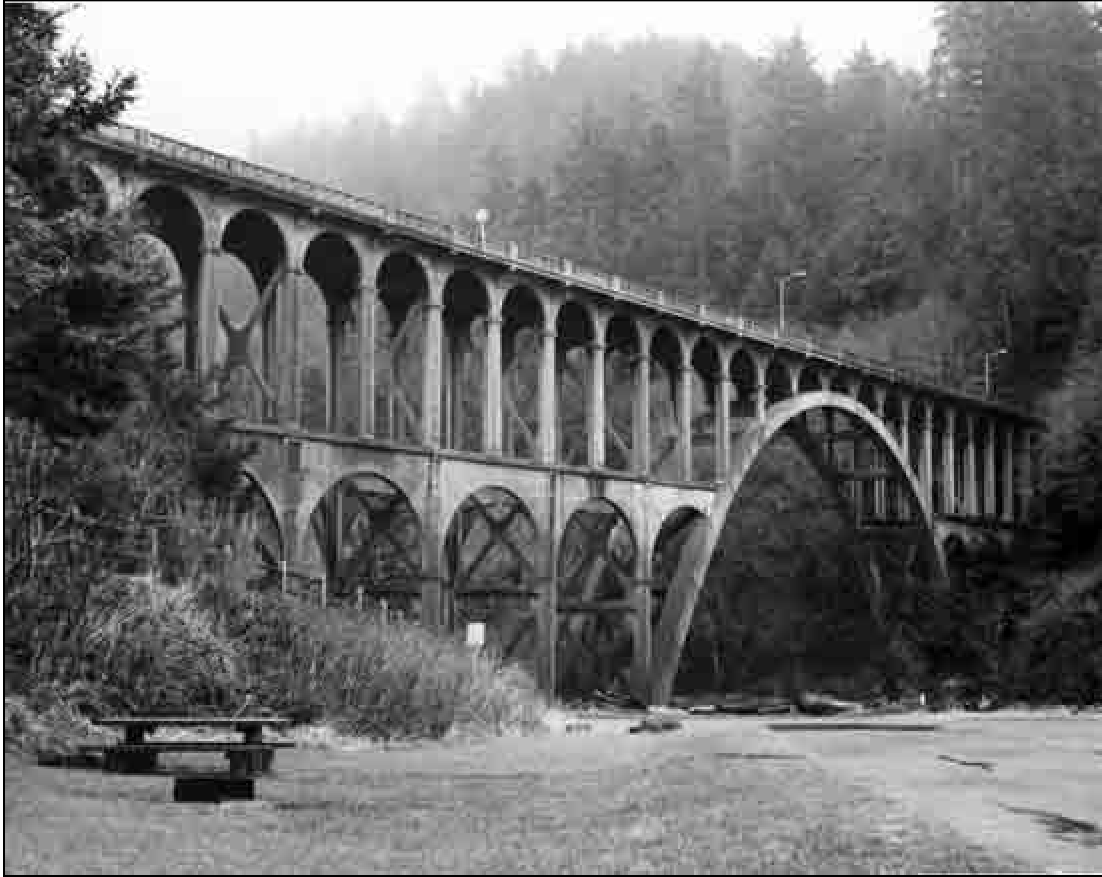
Structure Number 1113 Constructed – 1931 Oregon Coast Highway 9, M.P. 178.35 Reinforced Concrete Deck Arch Heceta Head, Lane County Ownership – State of Oregon
