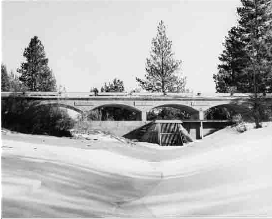
Structure Number 17C02 Constructed – 1914 Seismore County Road Reinforced Concrete Deck Arch Tumalo vicinity, Deschutes County Ownership – Deschutes County
