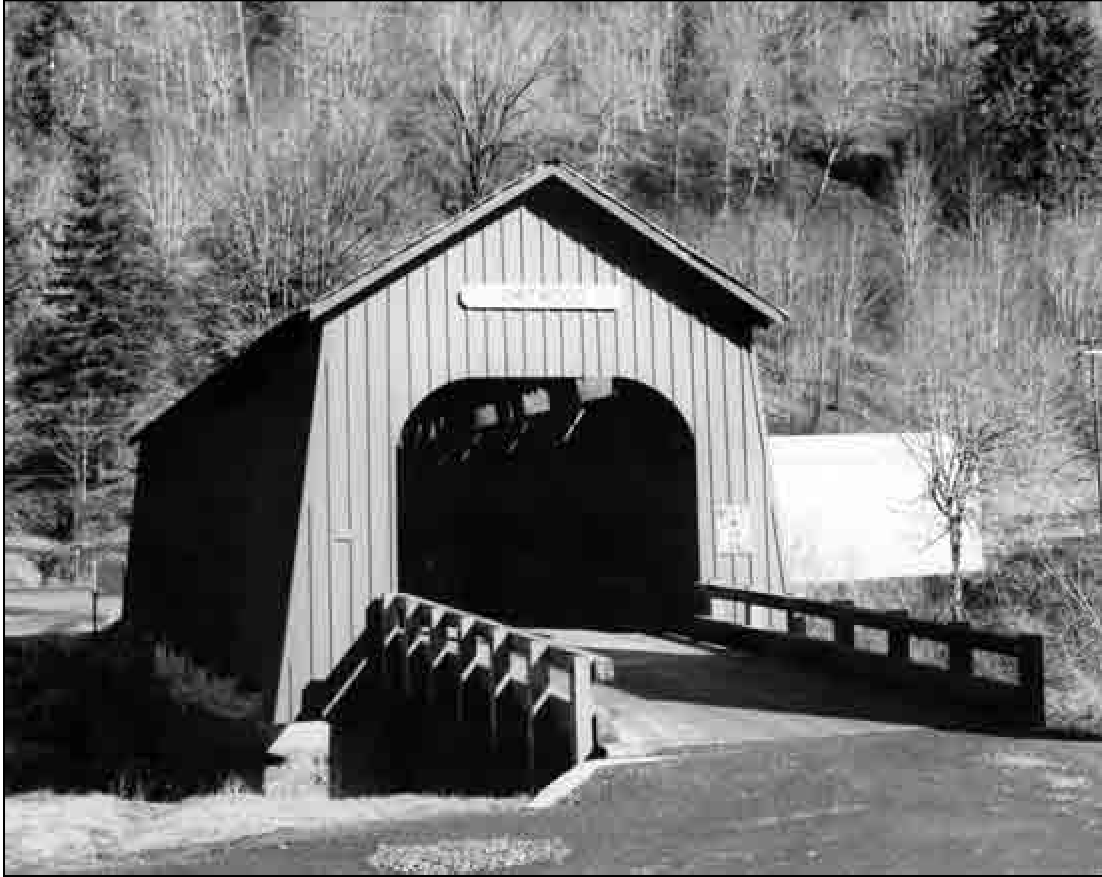
Structure Number 41C09 Constructed – 1926 Chitwood County Road 427, off the Timber Through Truss (Howe) Corvallis-Newport Highway 33, M.P. 18.11 Covered Bridge Chitwood, Lincoln County Ownership – Lincoln County
