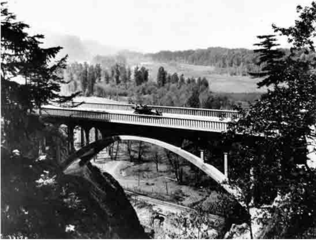
FIGURE 1. The Shepperd's Dell Bridge was constructed on the scenic Columbia River Highway in 1914 and was designed by the newly- created State Highway Department (1913). The structures on the Columbia River Highway established a tradition for excellence in design and compatibility with the environment.
