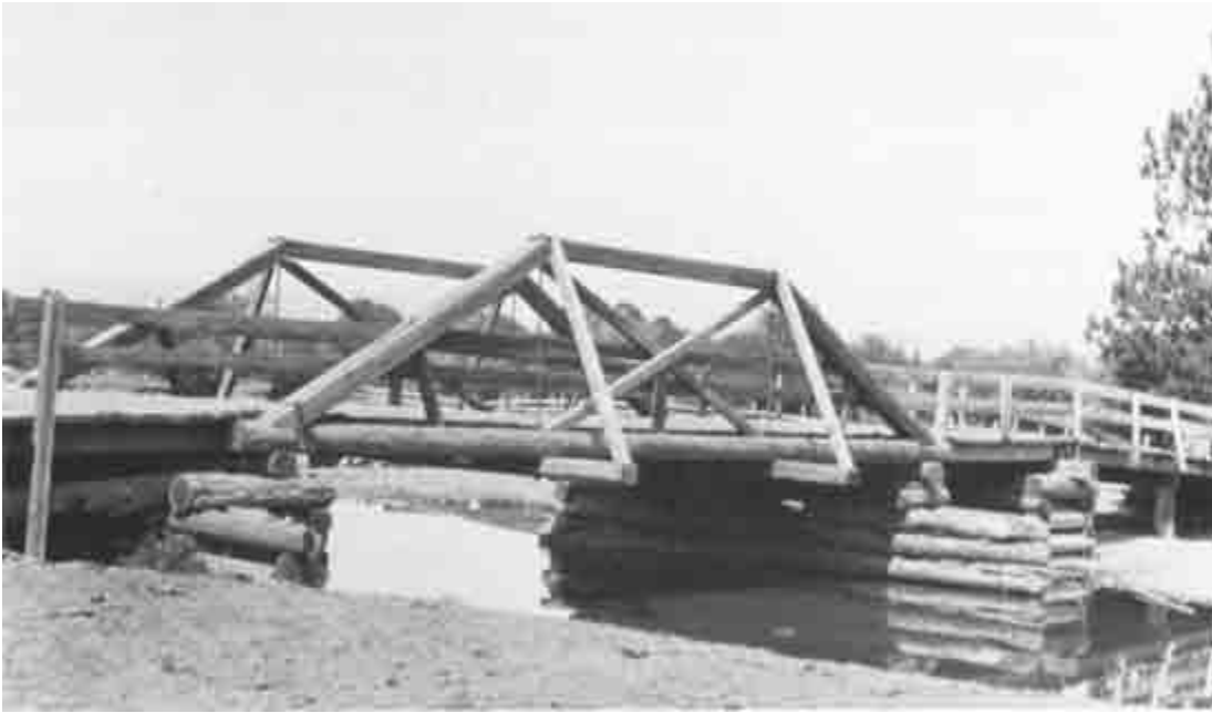
FIGURE 9. This timber and wrought iron queenpost truss is representative of early bridges in Oregon. Inexpensive, made of local materials, and constructed by local builders, these timber bridges were functional if not always long-lasting. (This bridge spanned Camas Creek near Ukiah, Umatilla County, and was built about 1900.)
