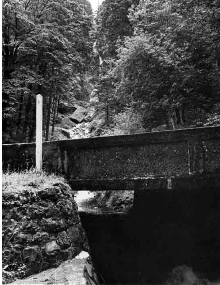
Structure Number 4533 Constructed – 1914 Crown Point Highway 125, M.P. 19.17 Reinforced Concrete Slab Multnomah Falls vicinity, Multnomah Ownership – State of Oregon County
