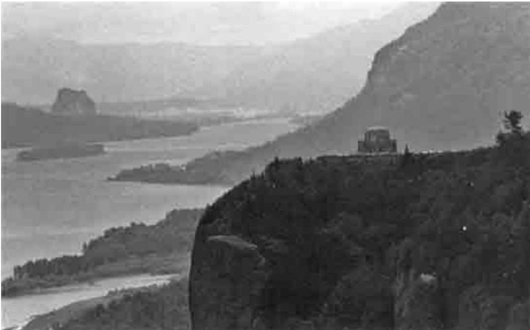
FIGURE 22. The 80-mile gorge of the Columbia River east of Portland posed an obstacle to highway building. Constructed between 1913 and 1922, the scenic Columbia River Highway was a major engineering feat. Crown Point Vista House, an observatory and rest area on the old highway, was completed in 1918.
