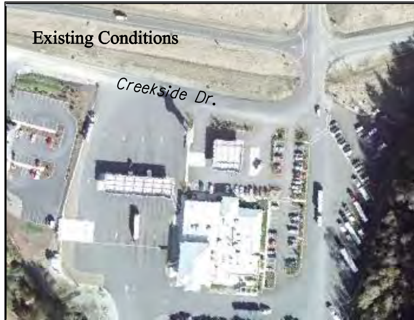
Figure: 8 Existing and Proposed access at Seven Feathers Truck and Travel Center
