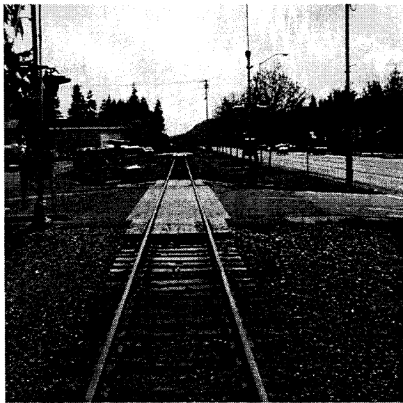
Maple Street (Facing South)
