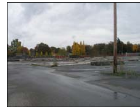
Existing Site Conditions
