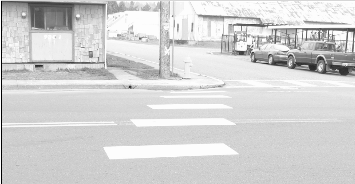
Figure 5 Crosswalk without Accessible Curb Ramp
