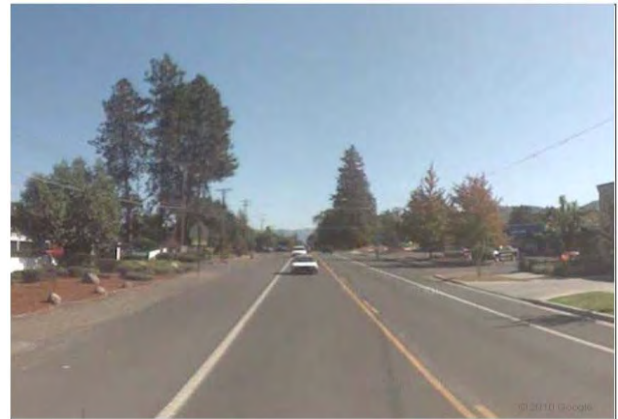
Siskiyou Boulevard – East of Walker Avenue Sidewalks and bike lanes on one side w/ shoulder bikeway other side
