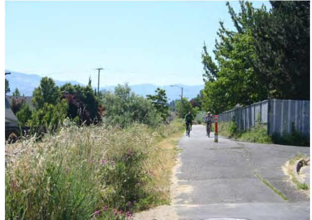
Exhibit 2-5: Multi-Use Path in Ashland
