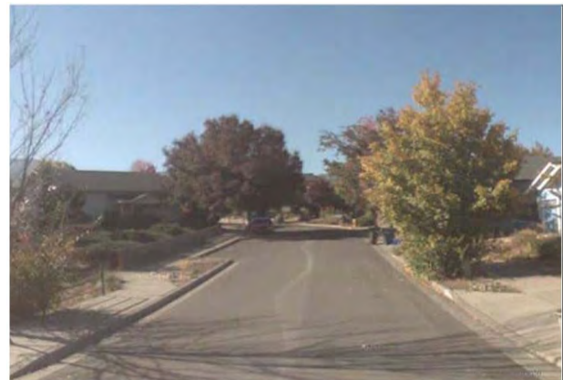
Crispin Street Sidewalks on both sides, Cyclists share roadway
