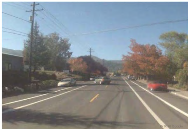
E Hersey Street – West of Carol Street Sidewalks on one side w/ on-street bike lanes
