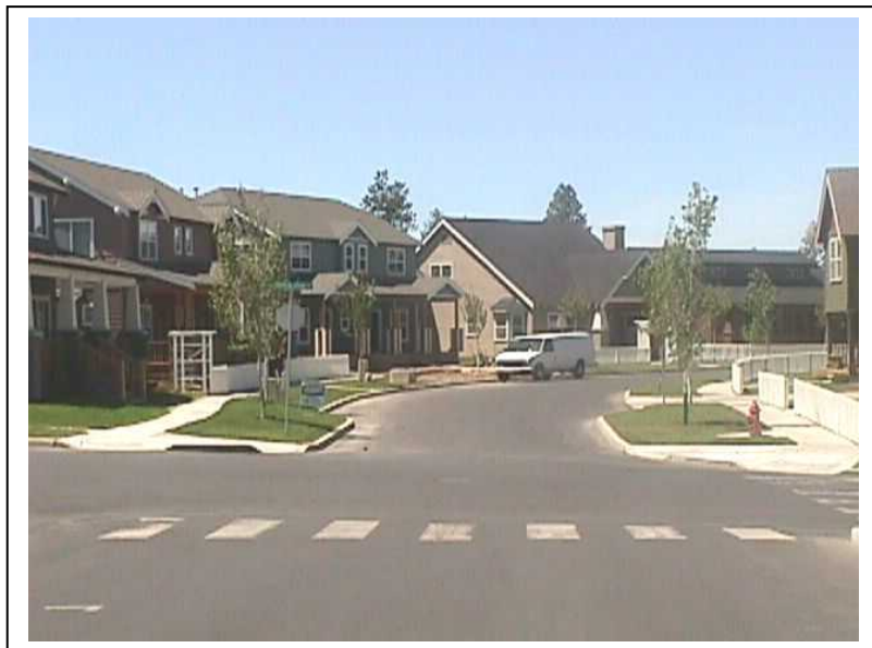
Figure 30. Example of a 20' wide curb extension or "choker" on a 30' wide street Photo by: City of Bend
