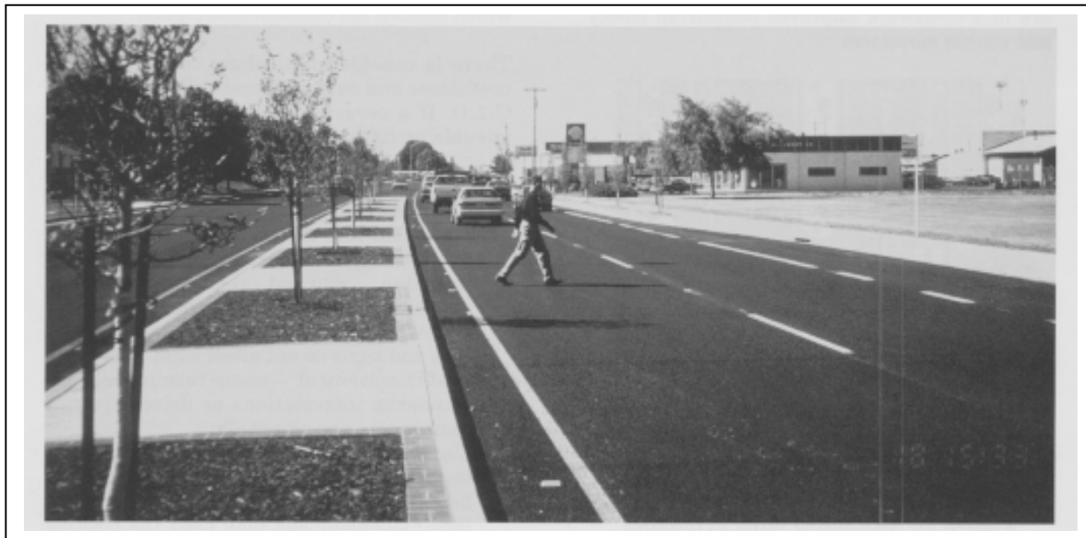
Figure 22. Median allows pedestrian to cross one direction of traffic at a time
