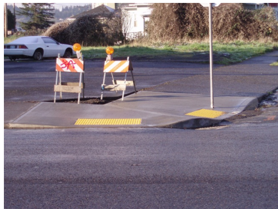
Figure 5-2. Dual Curb Ramps with Detectable Warning Strips
