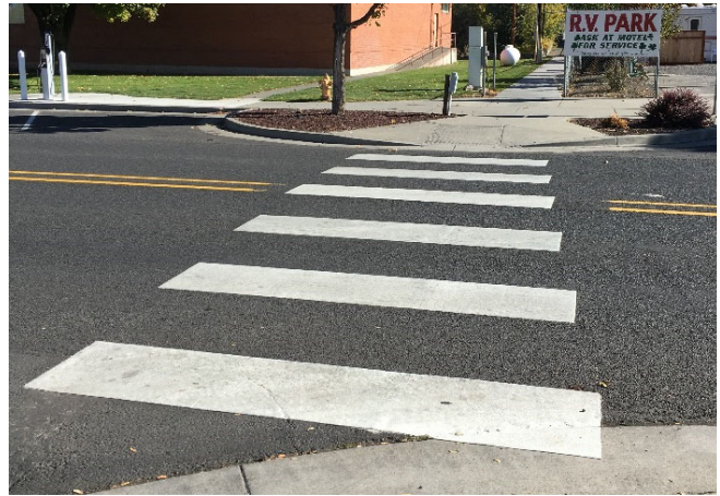
Example - Enhanced Crosswalk with Curb Extensions
