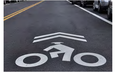
Example of a ‘Sharrow’ pavement symbol used to mark bike routes. Bicycles should travel over the ‘sharrow’ symbol. The placement, size and graphic design for sharrow marking can be found in current editions of the Manual for Uniform Traffic Control Devices (MUTCD). For neighborhood streets sharrows will typically be placed in the center of the travel lane.
