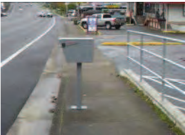
Though meeting ADA standards for passable width, the placement of mailboxes directly on the sidewalk may complicate travel for mobility-impaired pedestrians on Commercial Street.
