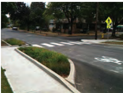
Curb extension with stormwater treatments on Rosemont Avenue NW
