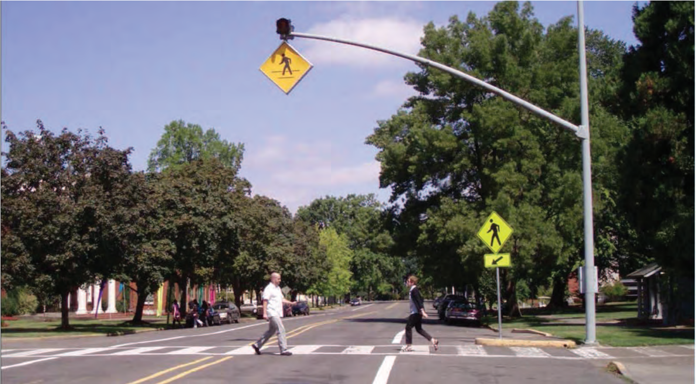
This mid-block pedestrian crossing on Winter Street includes high-visibility markings, signage and overhead warning lights.
