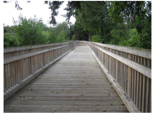
Example of a boardwalk
