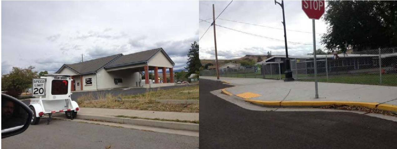
Exhibit 7 Speed reader board (left) and curb extension (right), both located near Union schools.
