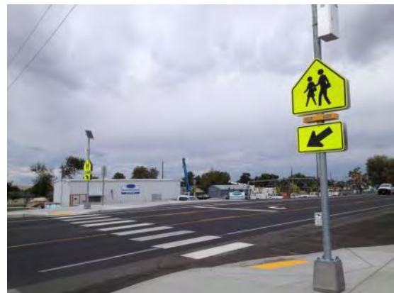
Exhibit 2 – Example of an RRFB (Irrigon, OR)
