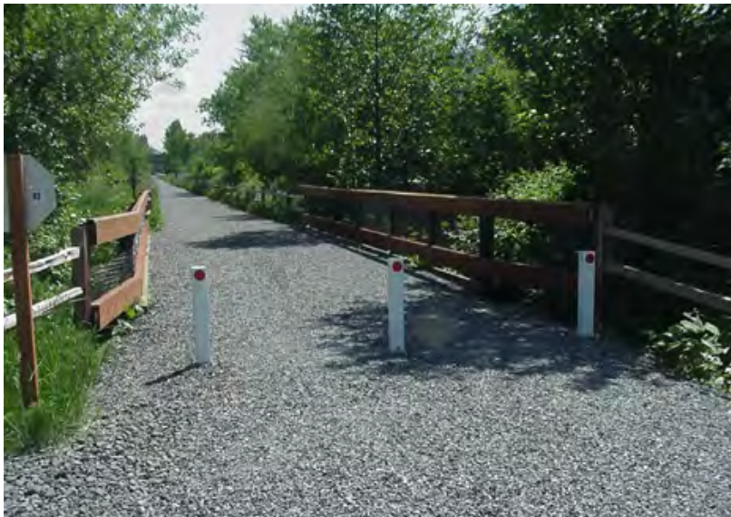
Soft-surface trails can be used by walkers, runners, mountain bikers, and equestrians, although there are safety concerns when horses share trails with other users. Soft-surface trails do not accommodate wheelchairs. Soft-surface trails cost less than paved trails to install, but have significantly higher annual maintenance costs.
