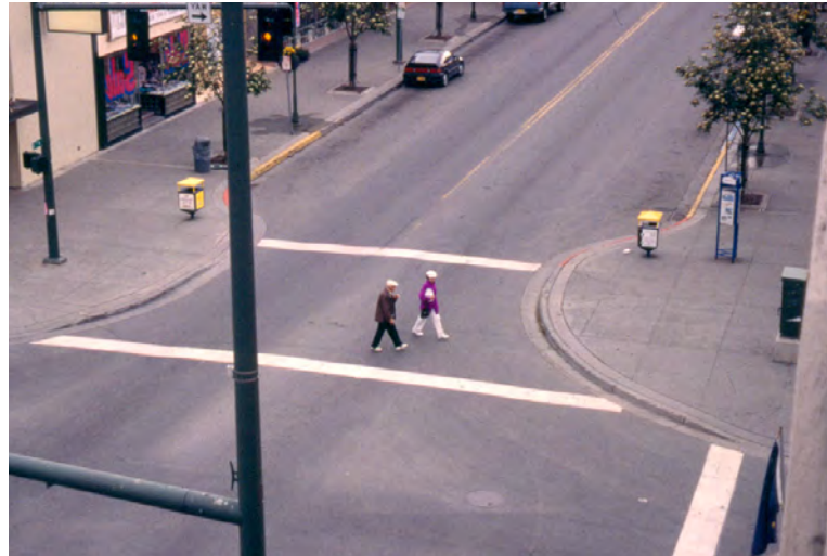
The intersection crosswalk shown has curb extensions on both sides of the streets—curb extensions shorten the required crossing distance and allow pedestrians to see around parked cars. Pedestrian signal heads and push buttons are also provided.
