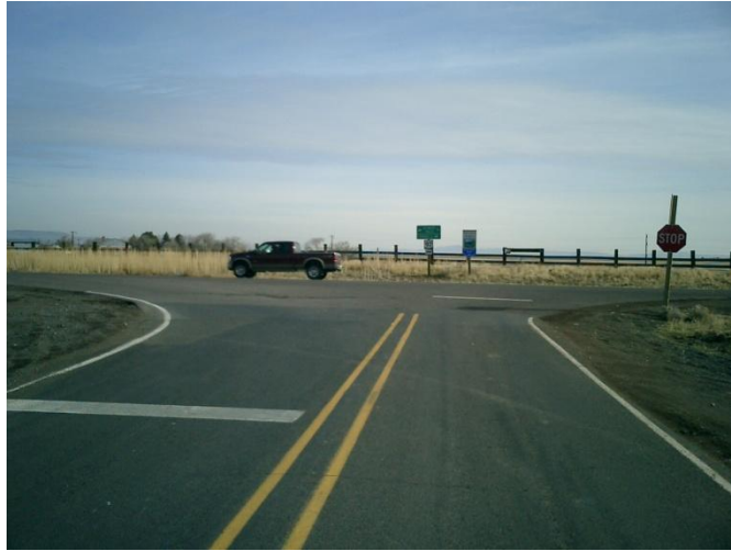
US 97 & Keno Worden Rd., from Keno Worden Rd. looking east
