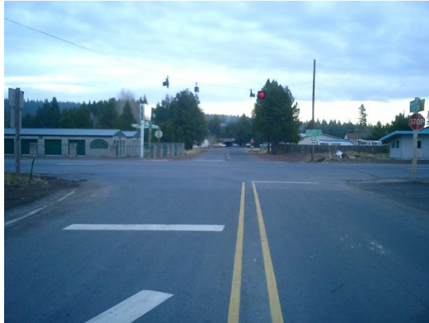
US 97 & Crescent Cutoff Rd., from Crescent Cutoff Rd. looking east
