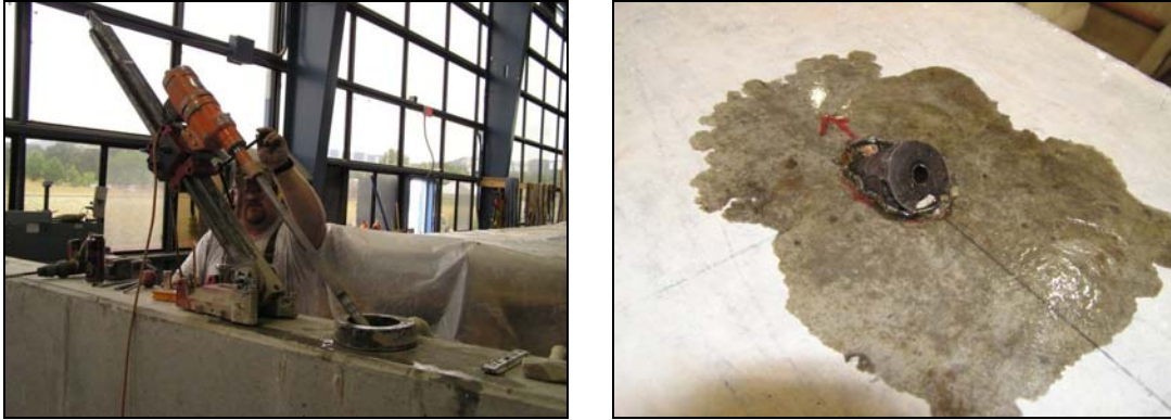
Figure 5.59: Internal stirrup installation
