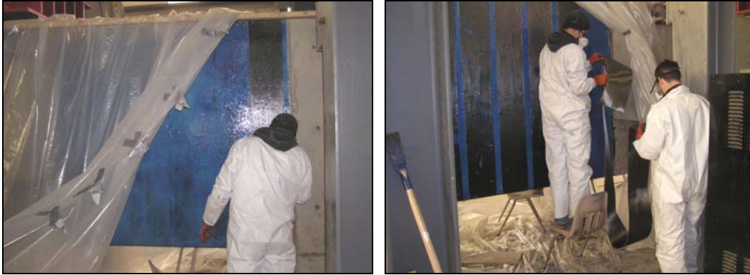
Figure 5.106: CFRP bent cap installation: strip installation
