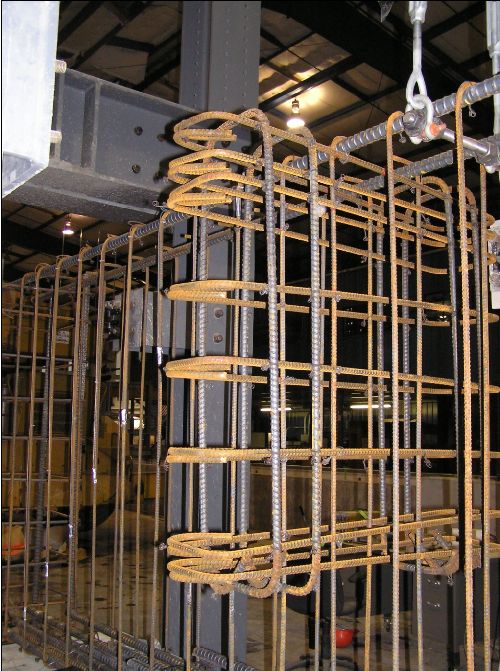
Figure 4.12: Typical bent cap stub girder assembly
