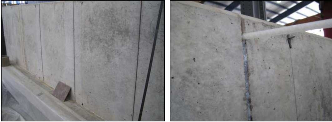
Figure 5.91: NSM installation: cut grooves (left) and initial epoxy application (right)
