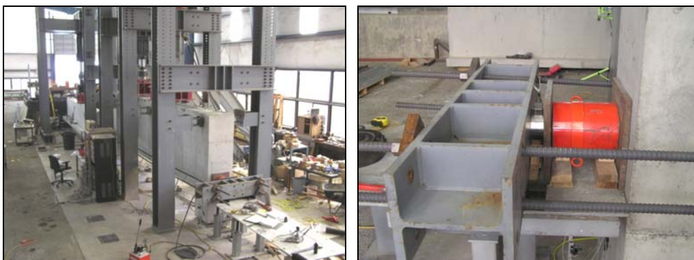
Figure 5.109: Post-tensioned bent cap installation
