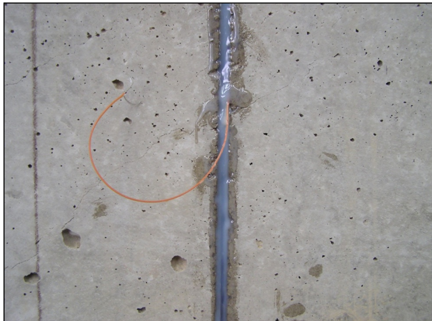
Figure 5.92: NSM installation: final product
