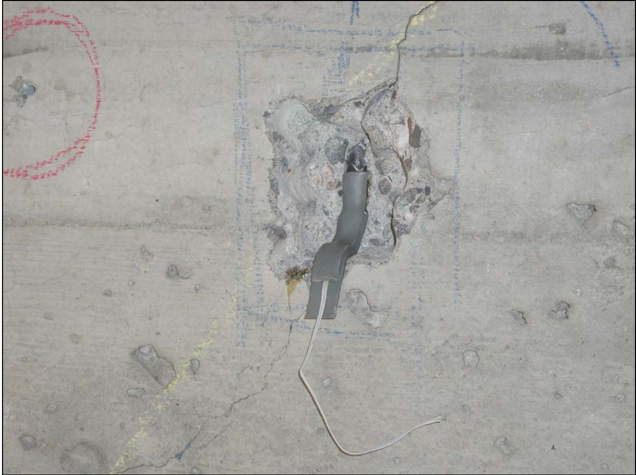
Figure 3.4: Example installation of strain gage on stirrup at diagonal crack location
