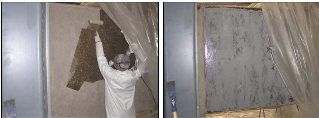
Figure 5.105: CFRP bent cap installation: primer (left) and putty (right)
