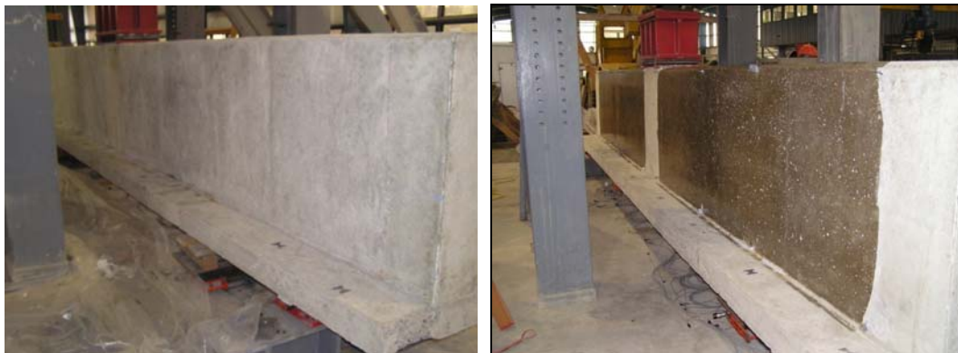
Figure 5.75: CFRP installation: ground surface (left) and primer application (right)
