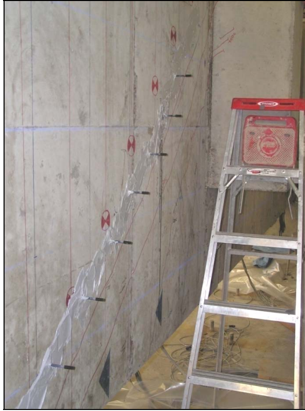
Figure 5.104: CFRP bent cap installation: epoxy injection
