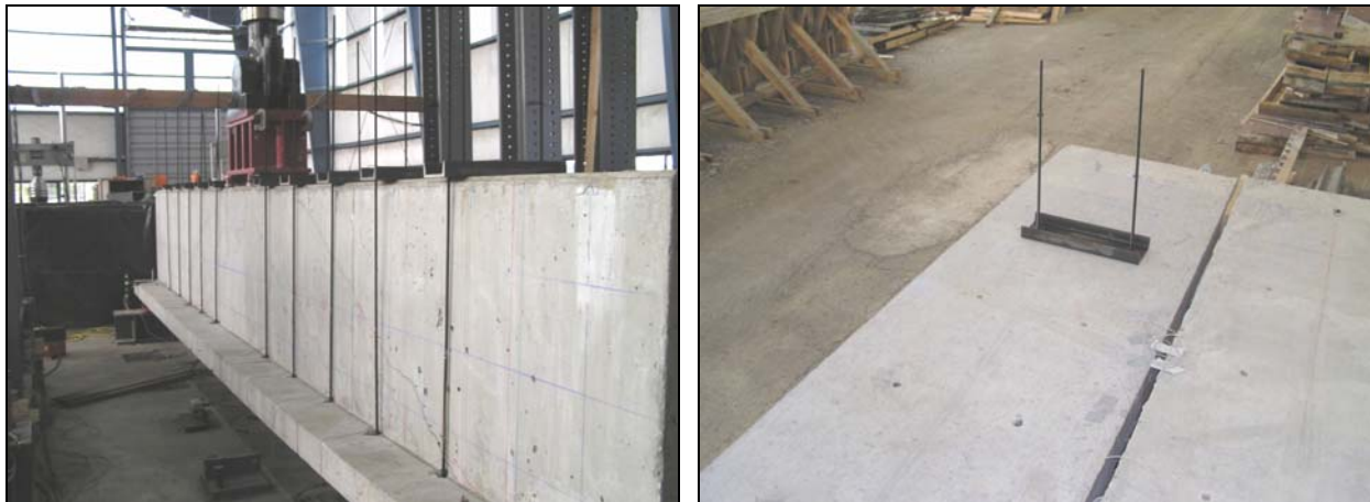
Figure 5.17: External stirrup installation
