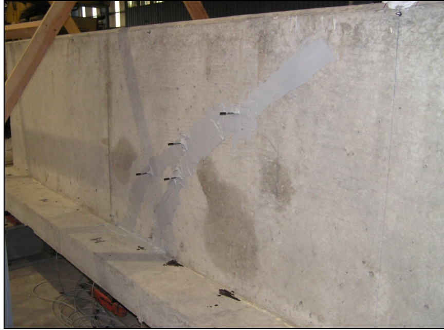
Figure 5.74: CFRP beam installation: epoxy injection
