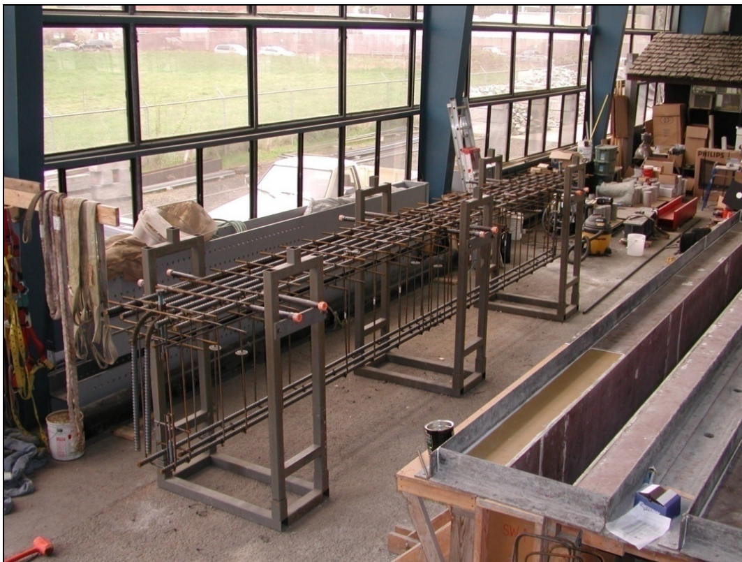
Figure 4.9: Assembly of completed reinforcing cage adjacent to formwork (IT specimen shown)
