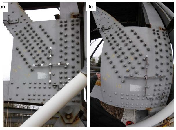
Figure 1.1: An image of a gusset captured by a) flat field lens b) fisheye lens. Note the downspout obstruction
