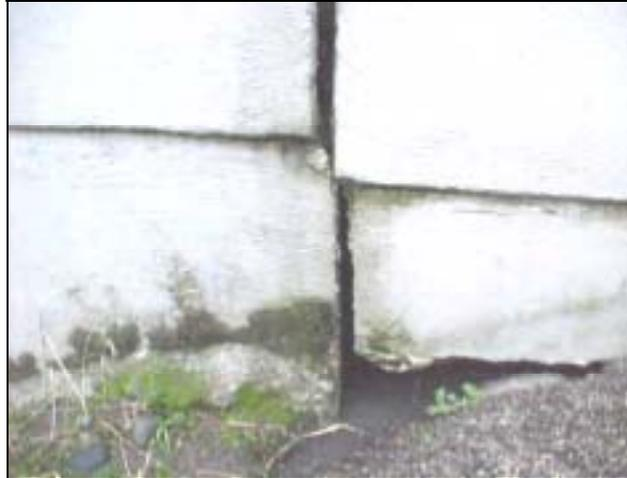
Figure 1.2: Side view of joint between the end panel and the adjacent slab before slab jacking
