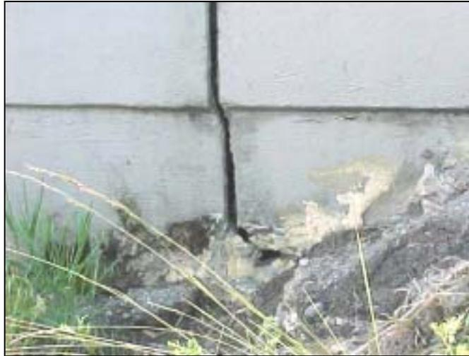
Figure 4.2: Side view of joint between the end panel and the adjacent slab after slab jacking
