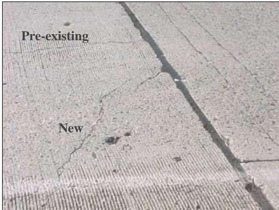
Figure 4.4: Cracks in the end-panel near Position 2
