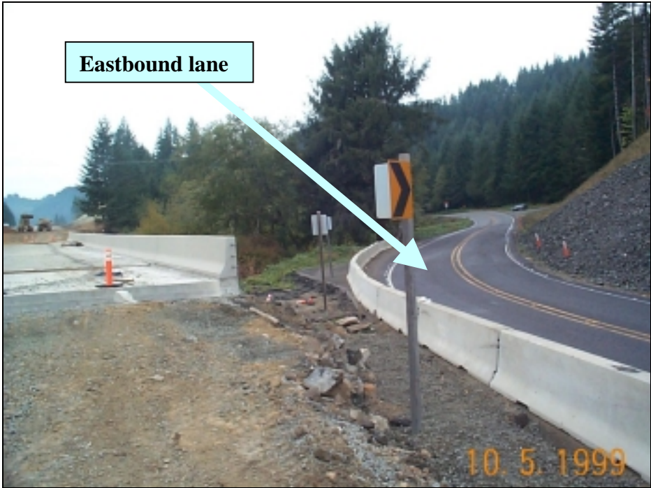
Figure 3.3: Project Site Looking West (New Highway Alignment is at Left)
