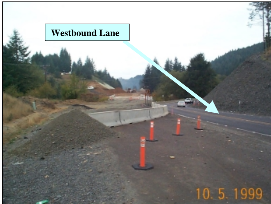
Figure 3.4: Project Site Looking West
