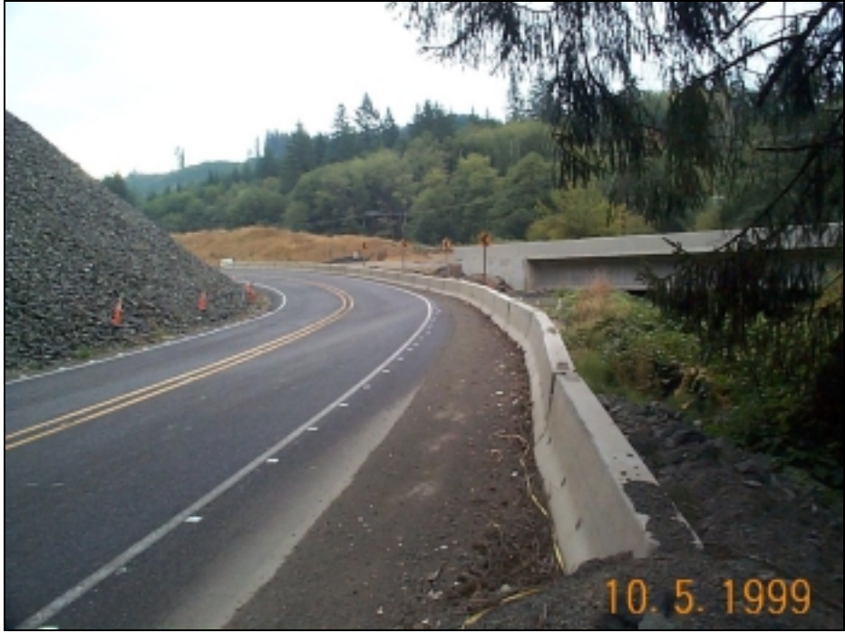
Figure 3.2: Project Site Looking East (New Highway Alignment is at Right)
