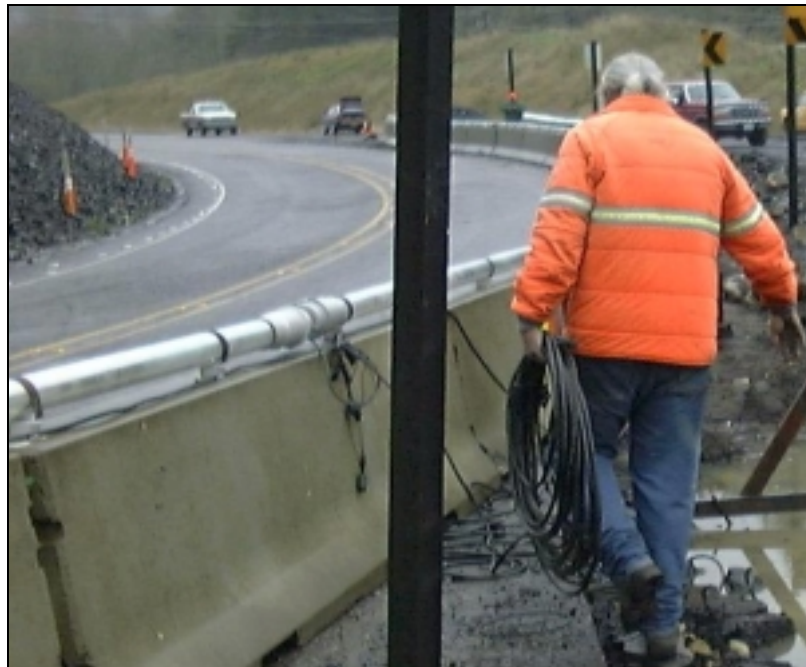
Figure 4.1: Installing the Connection Cable to the Lighted Guidance Tube
