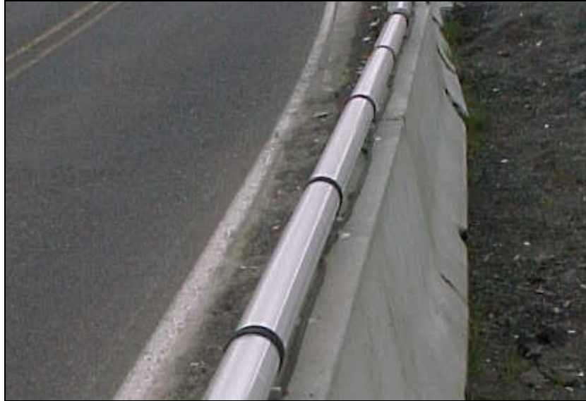
Figure 1.1: Lighted Guidance Tube Section
