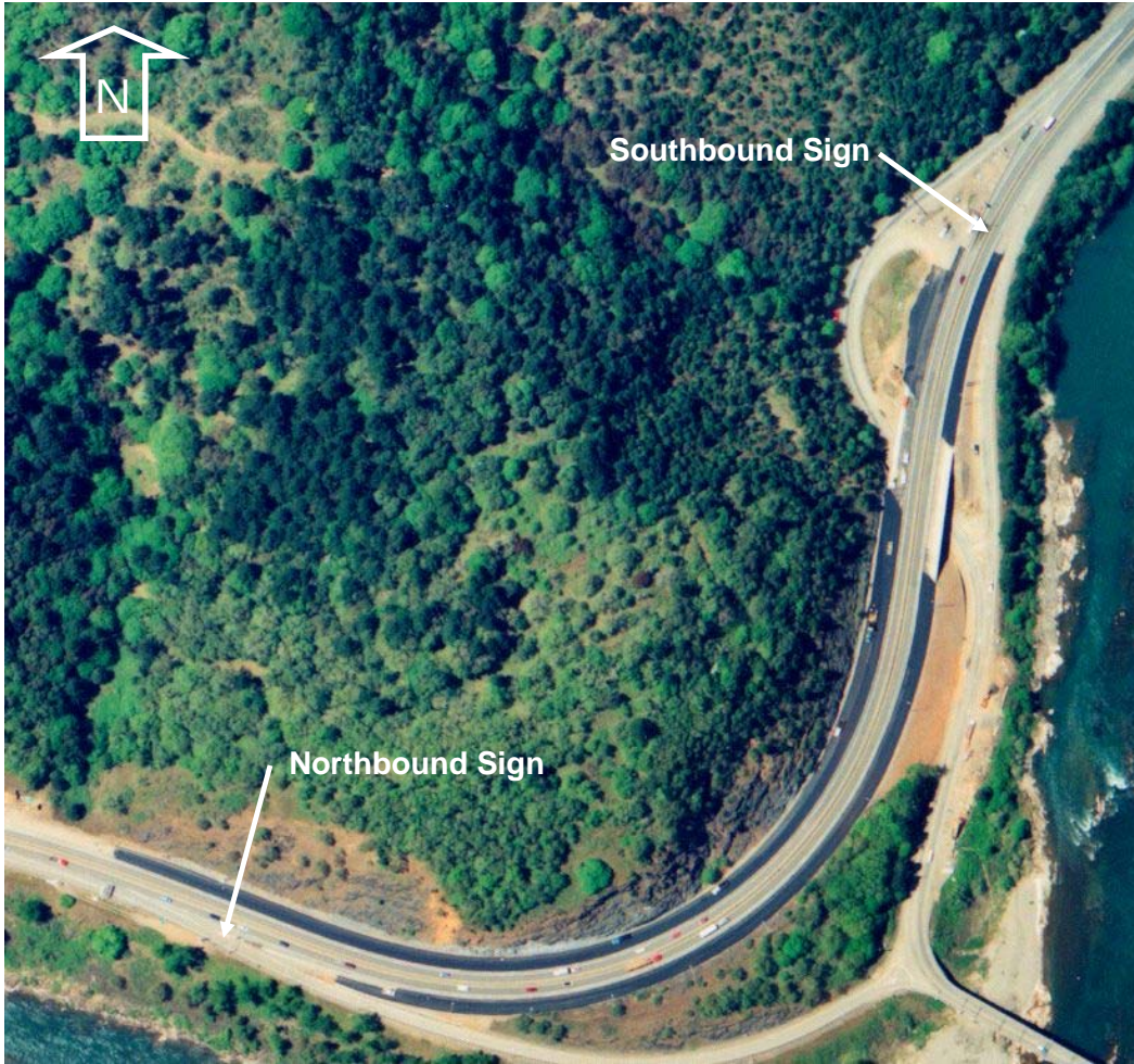
Figure 3.2: Aerial photograph of Myrtle Creek curves
