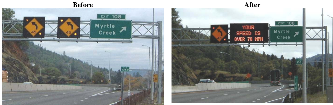
Figure 3.3: Northbound sign bridge, I-5 Milepost 108.00, before and after ACWS installation
