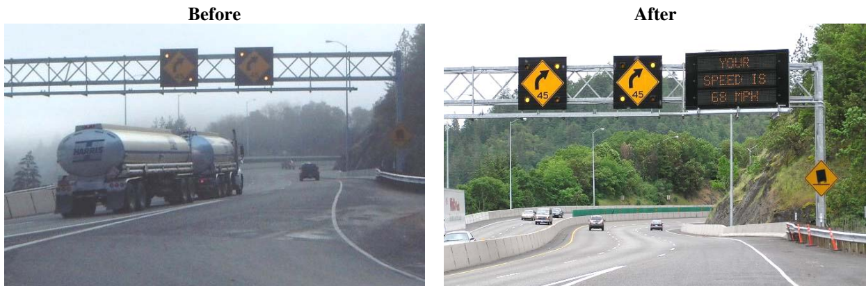
Figure 3.4: Southbound sign bridge, I-5 Milepost 108.35, before and after ACWS installation
