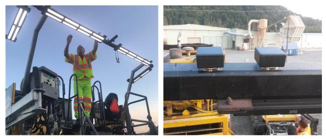
Figure 3.7: GPS sensor installation (left), and location on the paver light bar (right)
