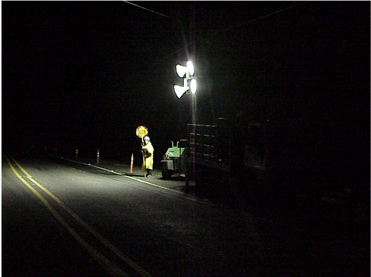
Figure 5.5: Orientation of light tower luminaires and illumination of flagger
