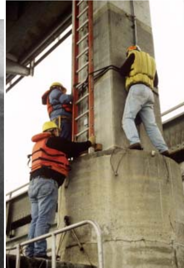
Figure 2.10: South column of pier 4, Richmond-San Rafael Bridge (CA), showing two of the four ICCP Zn anode bands (zones) and the SACP Zn anode zone on the barrel at the column base
