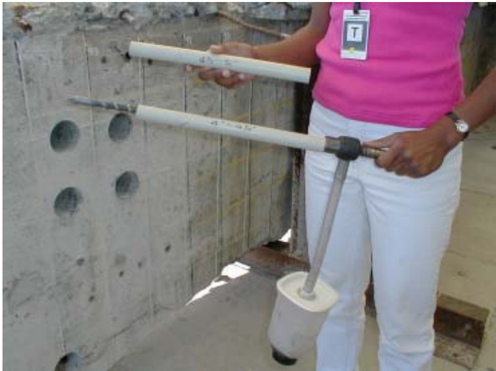
Figure 3.10: The hollow anchor drill bit, depth spacers, and vacuum filter assembly used in taking powder samples from concrete
