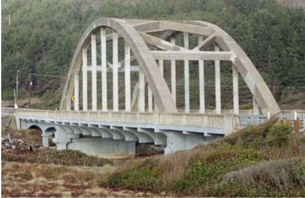
Figure 1.8: Big Creek Bridge built in 1931 and located on the Oregon coast south of Cape Perpetua
