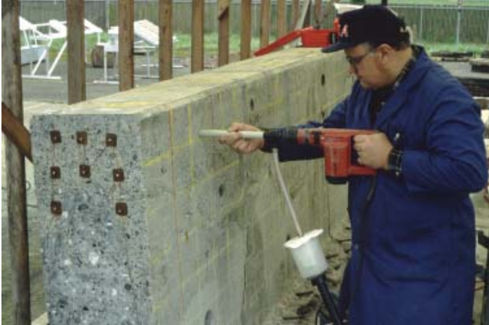
Figure 3.9: Concrete powder samples are taken from a concrete bridge beam using the Oregon DOT sampling equipment. Powder samples are analyzed to determine the salt concentration in the concrete as a function of depth in the beam.
