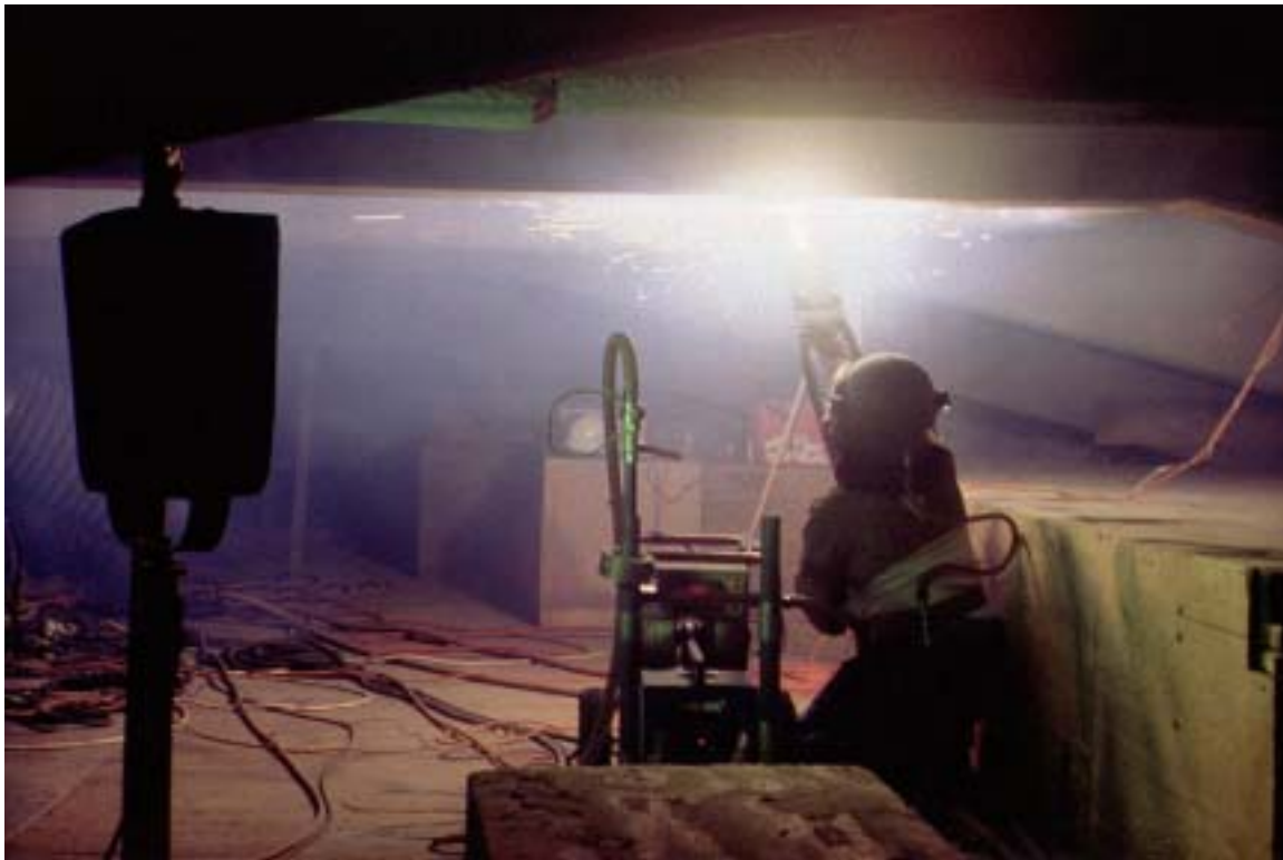
Figure 2.2: Thermal spraying Zn on a bridge substructure using the twin-wire arc-spray process
