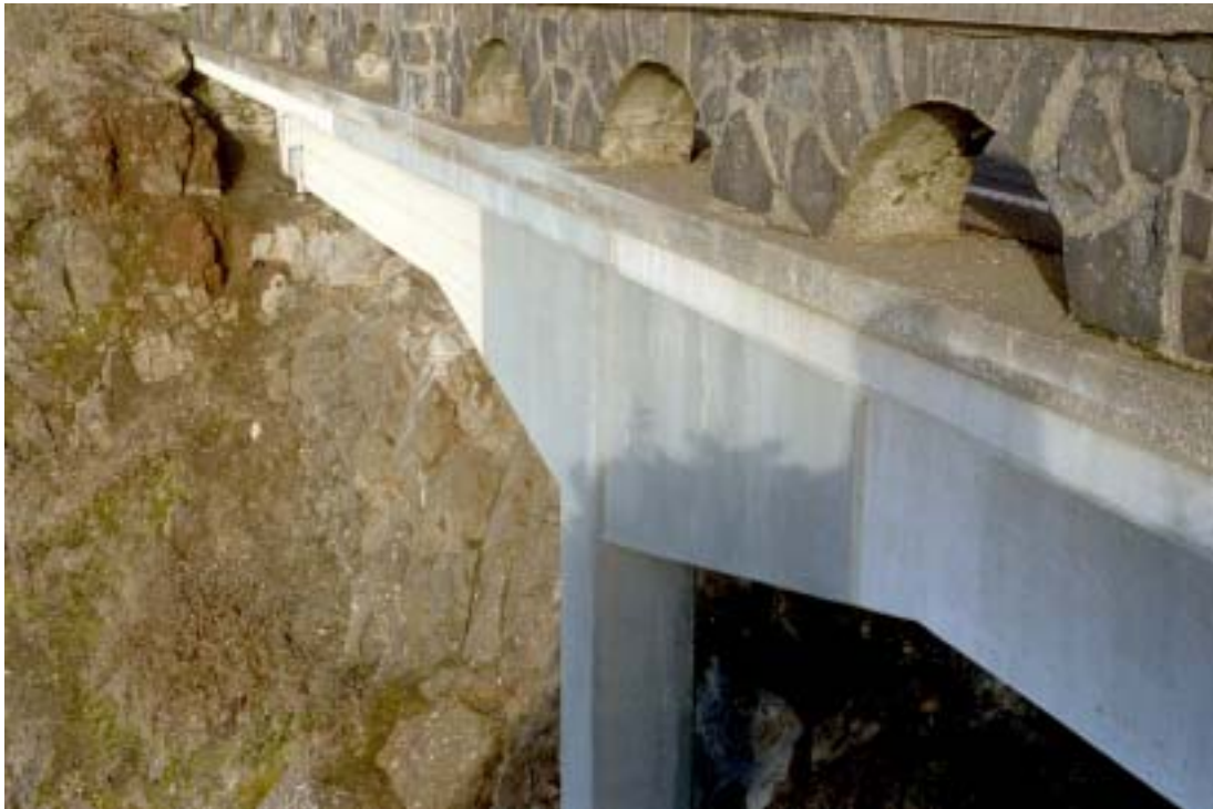
Figure 1.7: Cape Perpetua Half-Viaduct built in 1931 on the central Oregon coast
