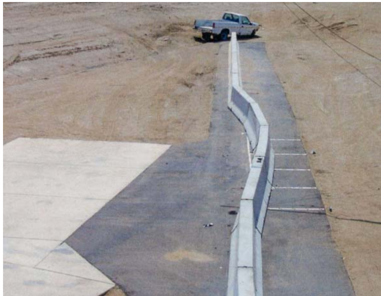
Figure 3.2: Standard F-shape barrier following Crash Test 1
