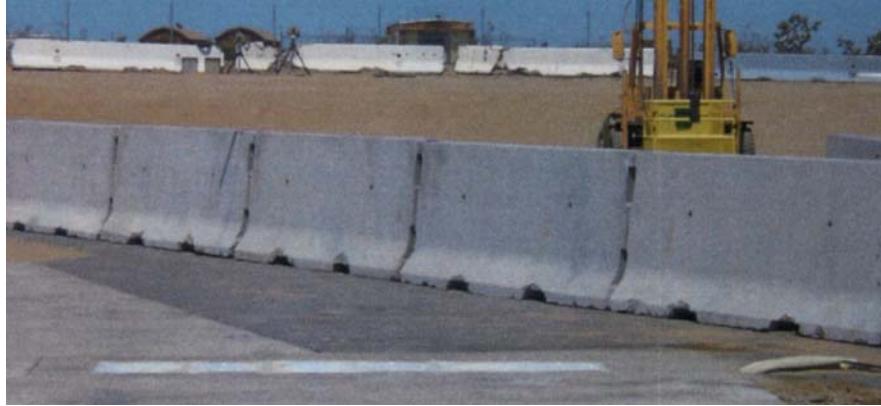
Figure 1.2: Tall F-shape precast concrete barrier
