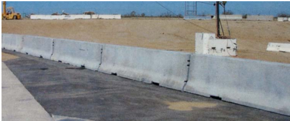
Figure 1.1: Standard F-shape precast concrete barrier
