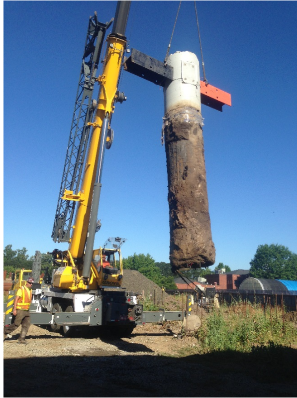
Figure 5.6: Picking of test shaft TDSFB from the post-test excavation.
