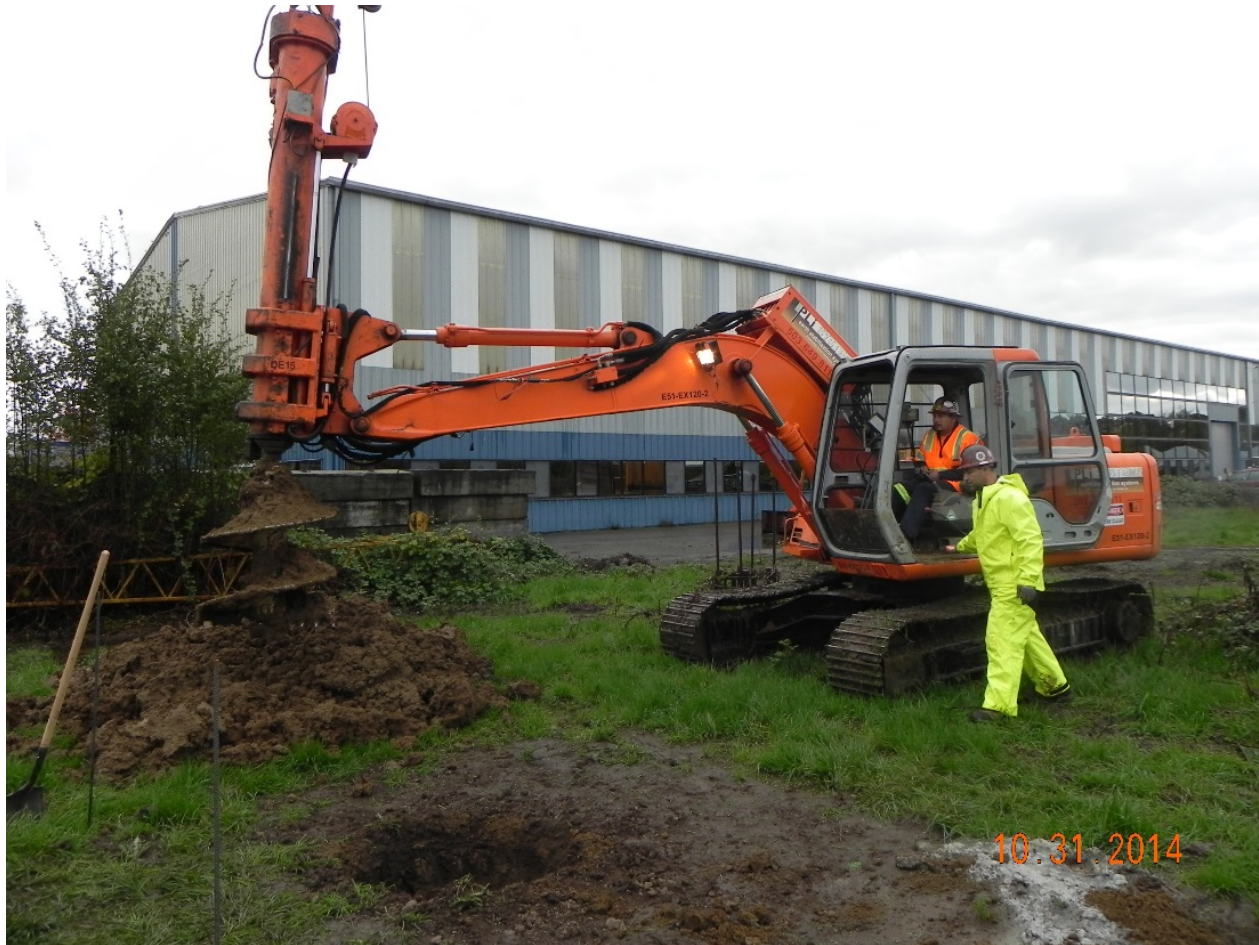
Figure 4.9: Excavating hole using excavator mounted drilling machines
