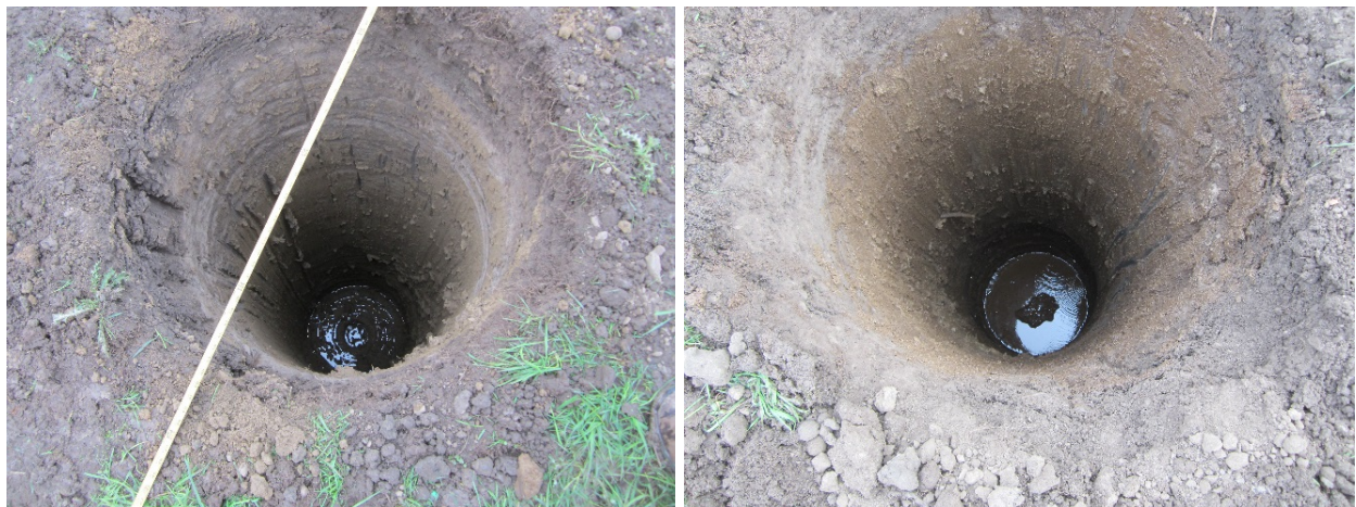
Figure 4.10: Drilled holes of (a) TDSFB and (b) TDS before the bottom was cleaned
