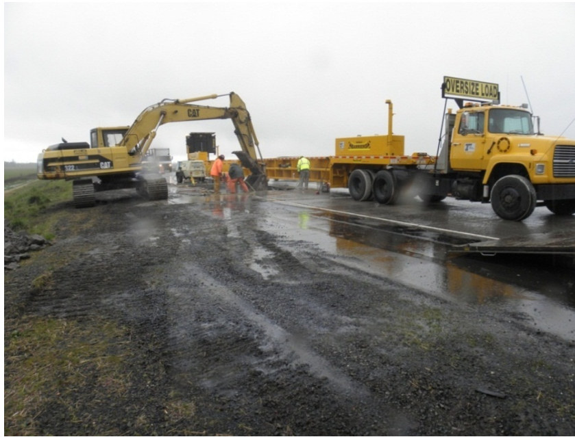
Figure 3.6: Workers Removing Concrete Pavement (Case Study #2)
