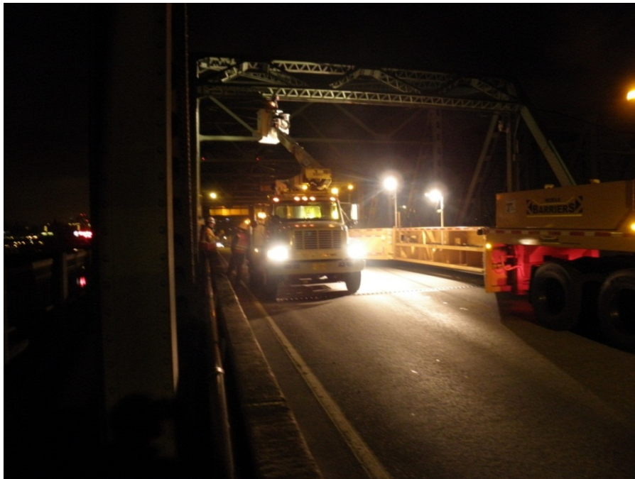
Figure 3.10: Workers Repairing Electrical Circuits on I-5 Interstate Bridge with MBT-1® (Case Study #3)
