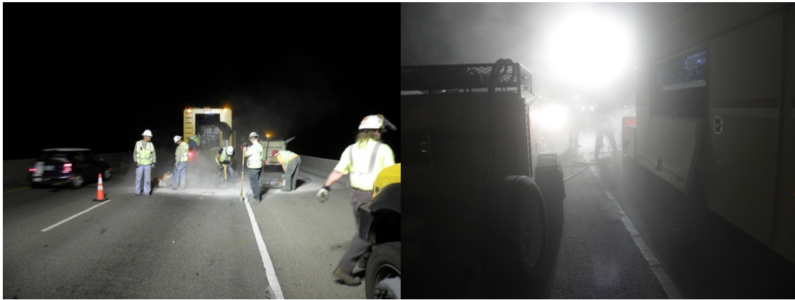
Figure 3.18: Jackhammering and Concrete Cutting (left); Dust from Concrete Cutter 'Fogging' Work Area (right) (Case Study #6)
