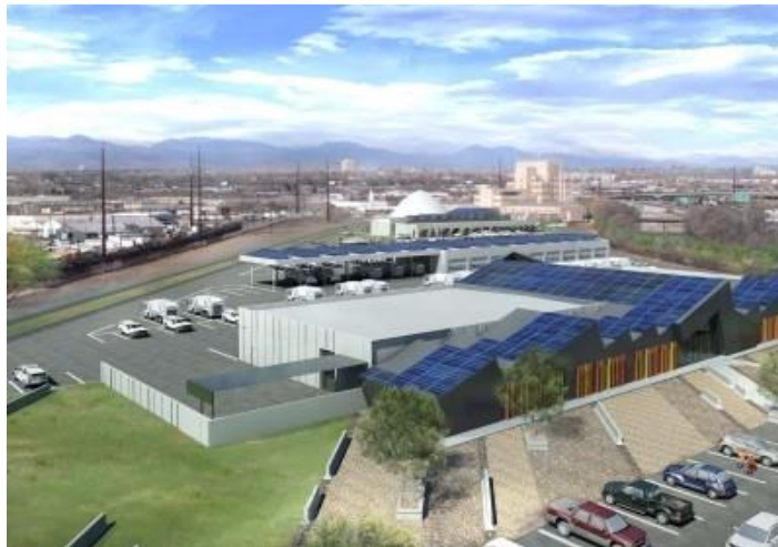
Figure 2.4. PV solar energy array installed at the City of Denver Public Works Department Central Platte Campus in Colorado (Lorand et al., 2013).
