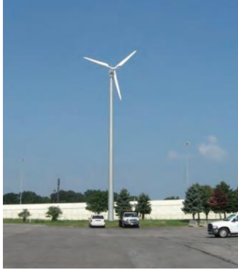
Figure 2.8. The 32-kW wind turbine at the Ohio Northwood outpost (Lorand et al., 2013).
