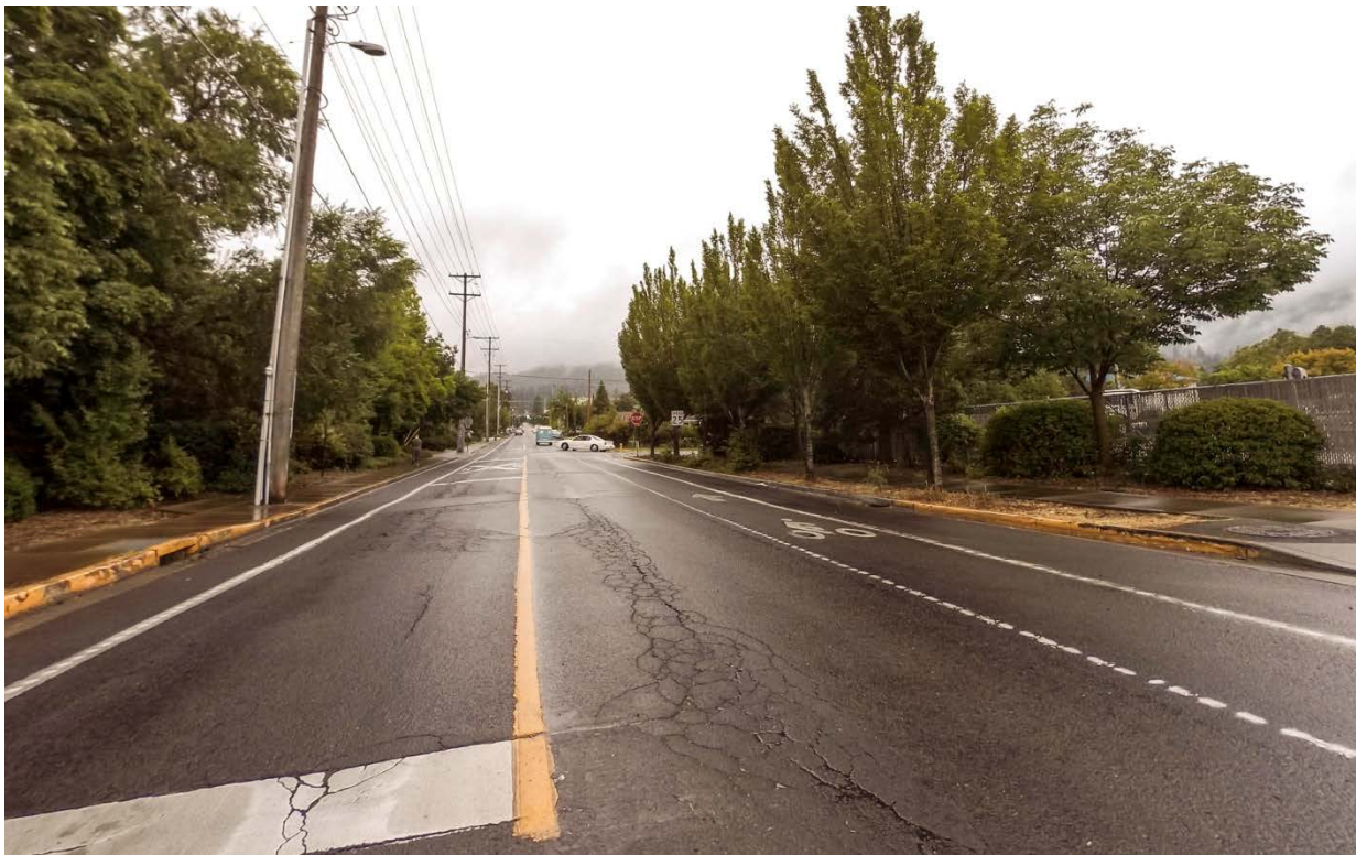
Figure 3.48: Bike facilities at the N Mountain Ave crossing
