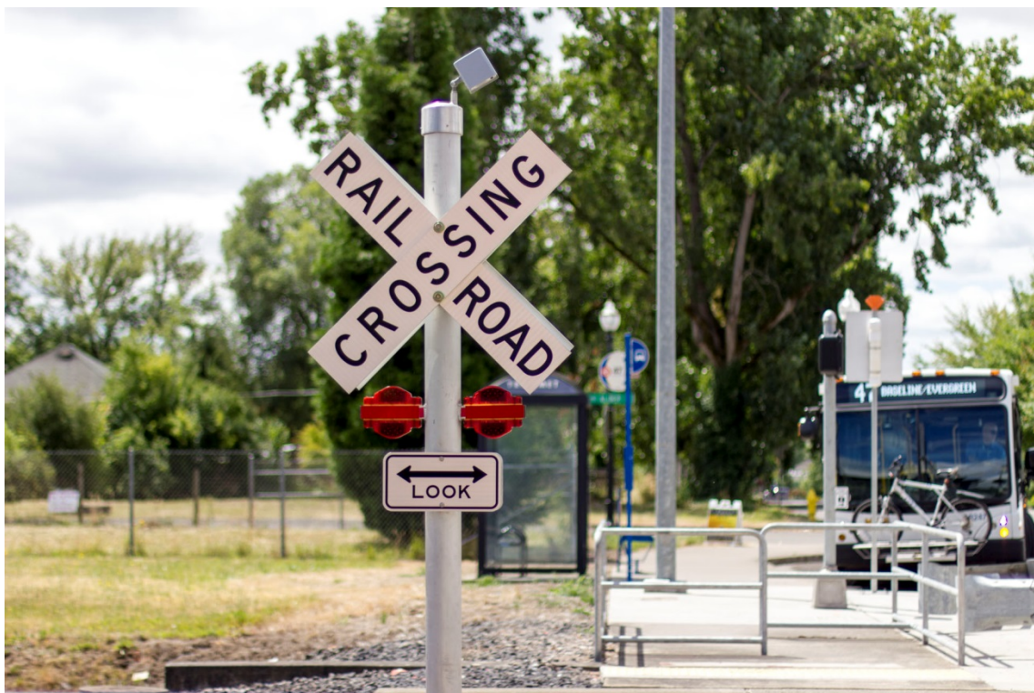
Figure 3.12: Active TriMet Style Pedestrian Flashers (TMPF's) and pedestrian fencing
