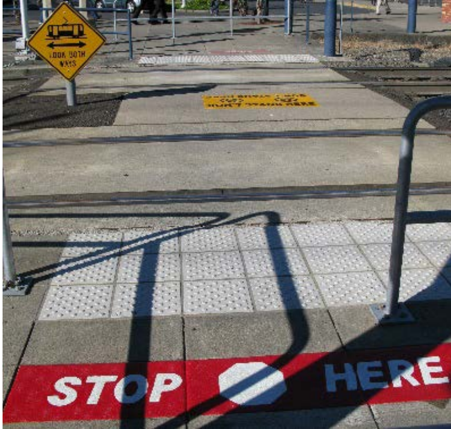
Figure 5.16: Pavement Marking (N/A, N/A)
