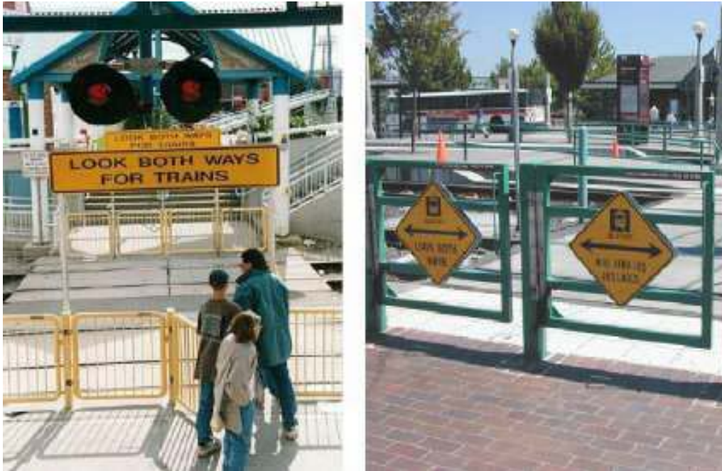
Figure 5.34: Pedestrian Manual Gates, (Korve, Hans W. , Jose I. Farran, Douglas M. Mansel, et al., 1996)
