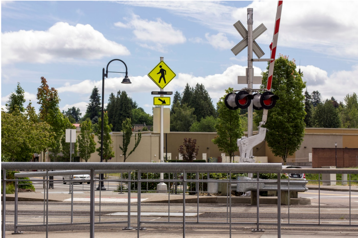
Figure 3.3: Active and passive treatments at the NW Civic Dr crossing
