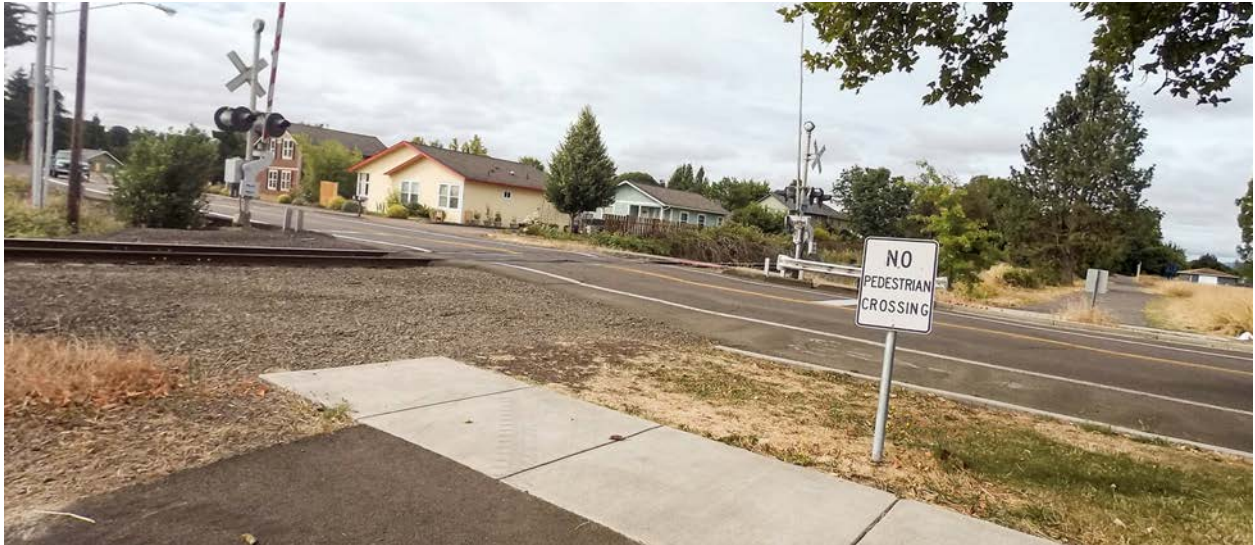
Figure 3.35: The sidewalk suddenly stops at the tracks
