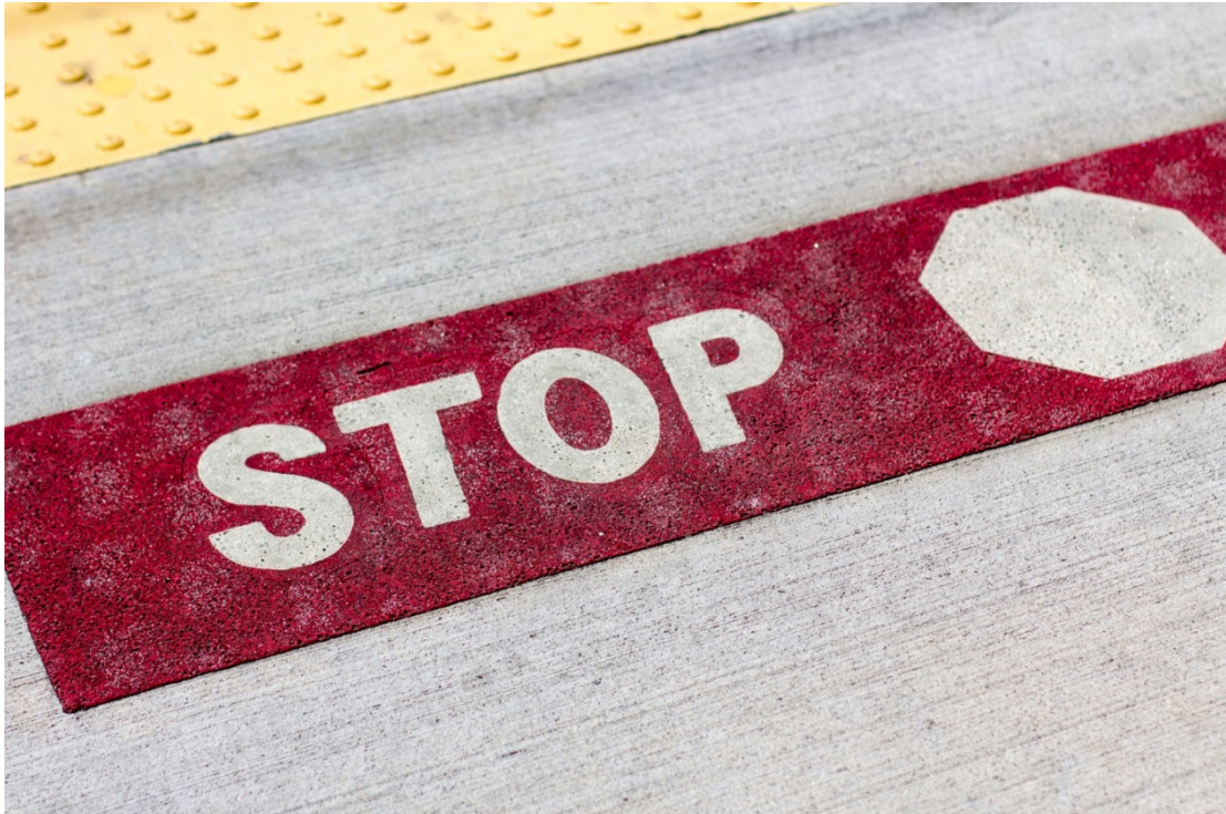
Figure 3.11: Tactile surface and painted stop signs for pedestrians
