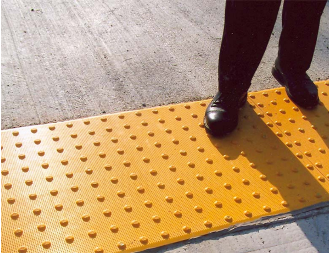
Figure 5.17: Tactile Warning (N/A, N/A, N/A)
