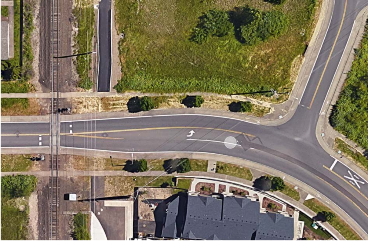
Figure 3.39: Satellite photo of the Walnut Blvd crossing in Corvallis, OR (Google, 2016) (Trail is marked in orange)
