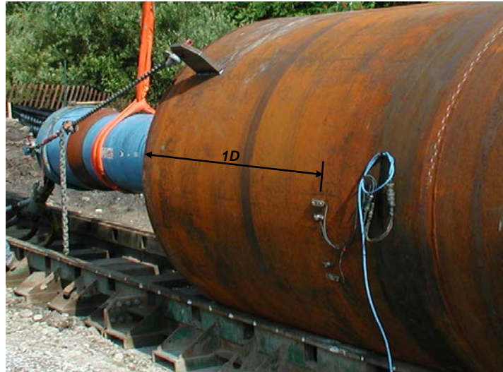
Figure 3.9 Two pairs of accelerometers and strain gages mounted to the pipe.
