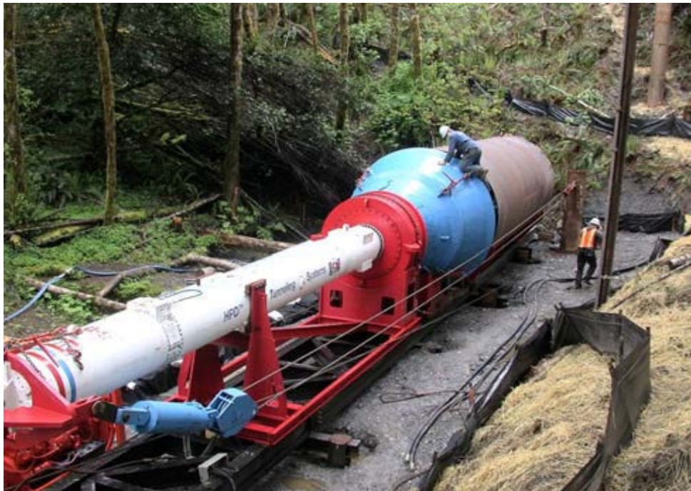
Figure 2.7: Hydraulic Hammer driving 3050 mm diameter pipe (after Piehl 2005).
