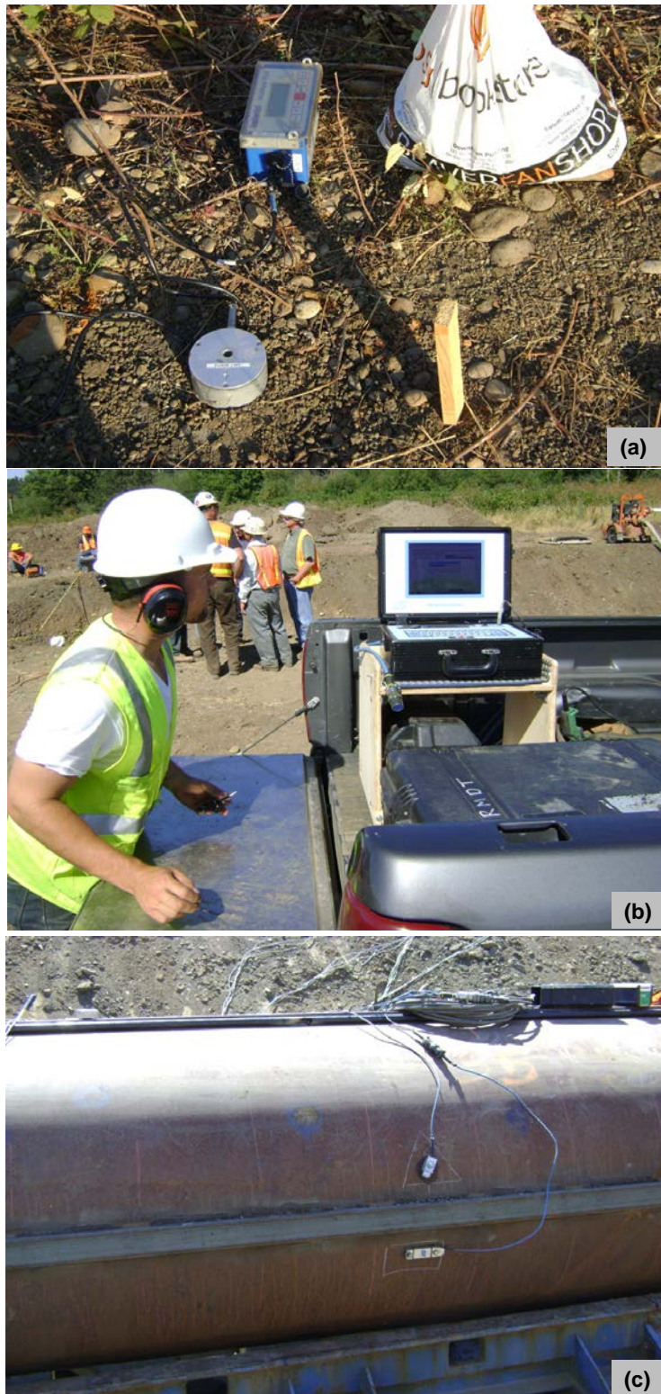
Figure 3.30: Photos showing field instrumentation: (a) Minimate Plus seismograph with standard geophone and a sandbag (b) Pile Driving Analyzer (PDA), and (c) high frequency strain gauges and accelerometers attached to the pipe.
