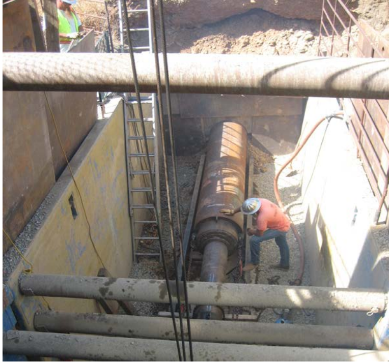
Figure 3.17: Pipe ramming in progress for 760 mm casing installation ( Bennett Trenchless 2010a ).
