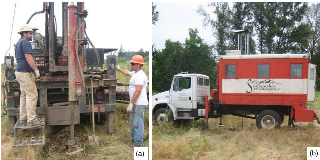
Figure 3.22: In-situ testing at the site including (a) Standard Penetration Testing (SPT) , and (b) Cone Penetration Testing (CPT).
