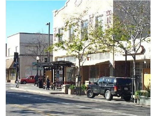
ABOVE: A bus stop bump-out creates a safe haven for waiting. Parallel parking fits before and after the stop. Photo credit: E. Rosenberg
