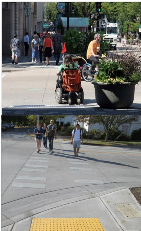
ABOVE: Improvements such as no-slip strips, crosswalk striping, and landscaping are small enhancements that add great value when connecting people to transit. Photo credit (bottom): City of Corvallis
