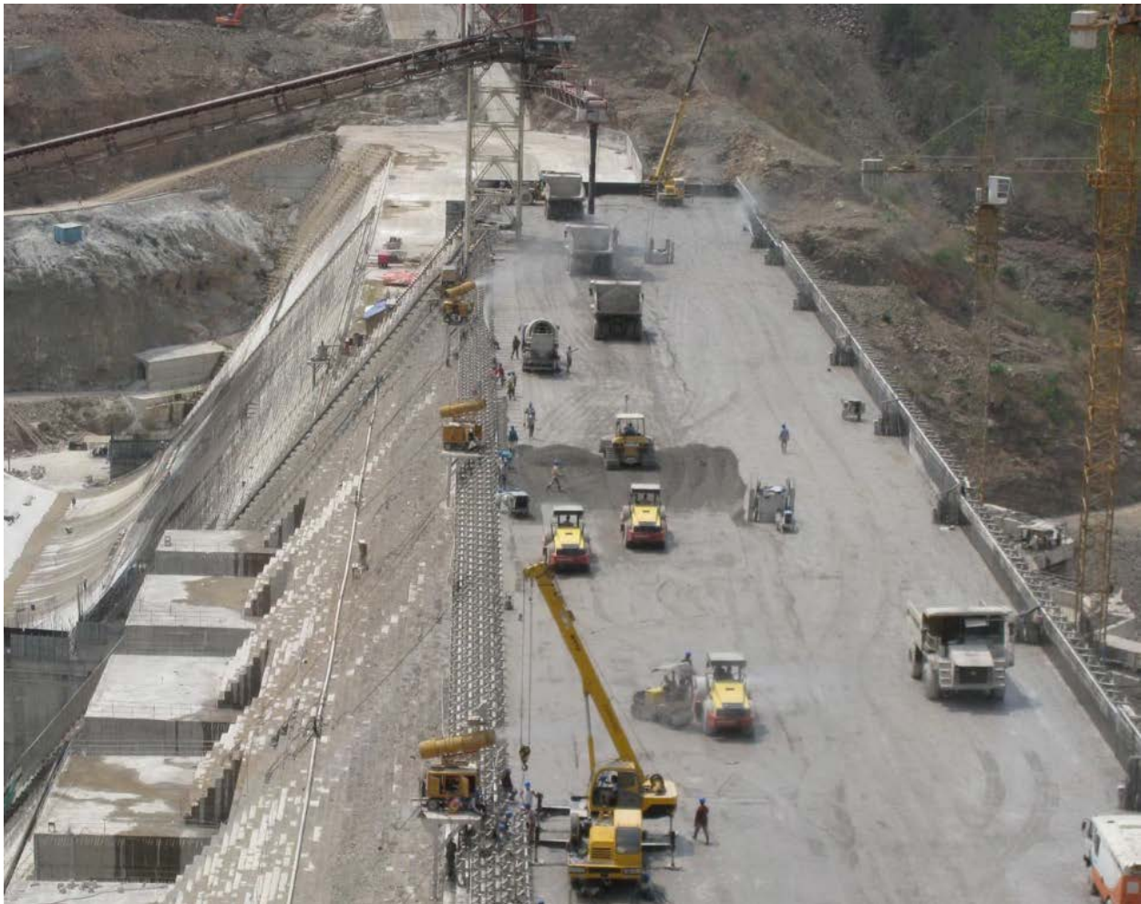
Figure 3-1. Typical RCC Dam Construction Pine Creek Dam Concept Study
