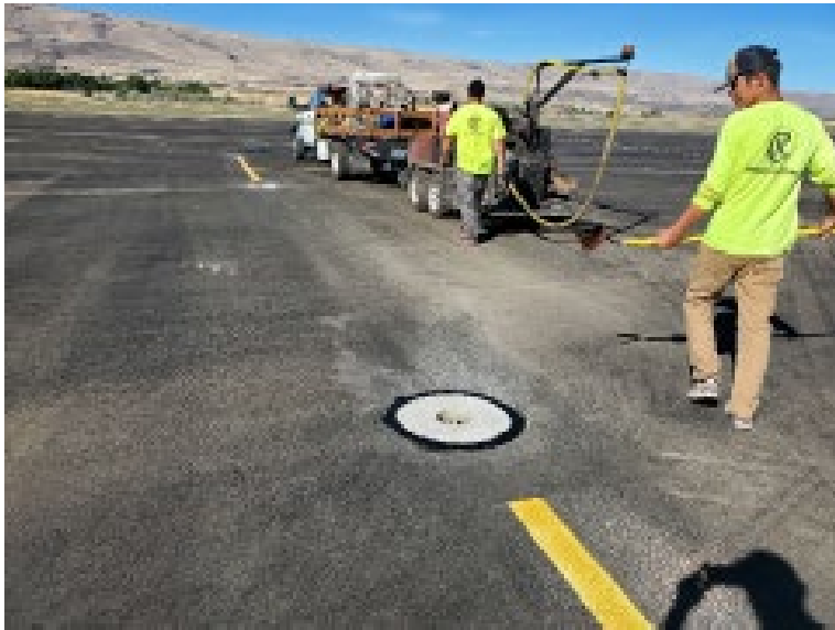
Columbia Gorge Regional Airport 2019 – North Apron Reconstruction
