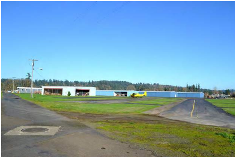
Photo 19. Historic-period T-hangers were once located at the concrete pads where the plane at center is parked. The view is facing northeast from South Airport Road.
