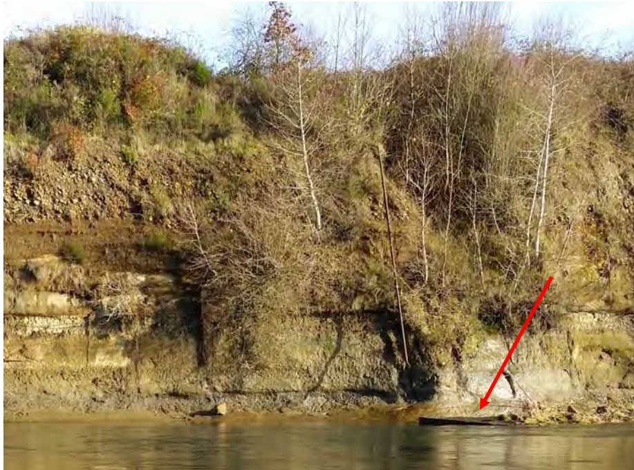
View of concrete railroad trestle remnant (denoted by red arrow) near the north bank of the Molalla River and the downgrading trench opening to the former bridge approach at 17/2634-1. The view is towards the northeast.
