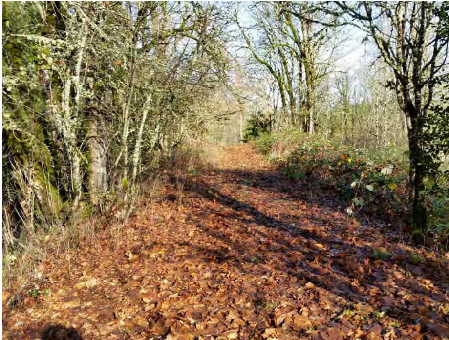
Remnant railroad grade on raised berm on the south side of the Molalla River at 17/2634-1. The view is towards the north.
