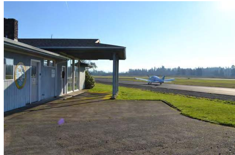
Photo 16. A Pilot Lounge/Airport Office constructed circa 1968 is located adjacent to a modern taxiway used in association with Runway 14-32. The view is facing south.
