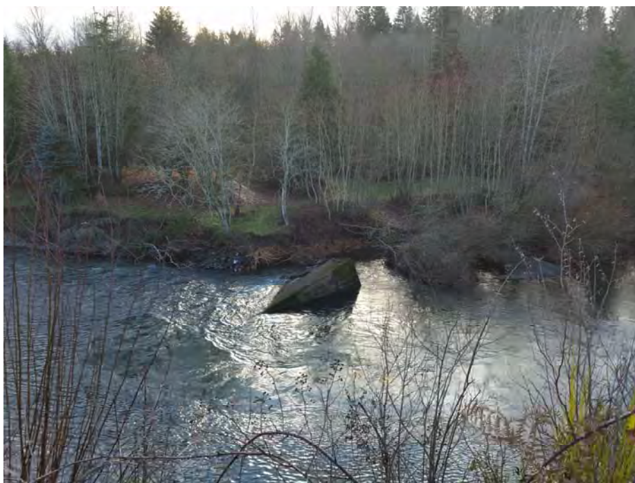
View from area of former trestle approach looking south across the Molalla River along the former alignment of the Willamette Valley Southern Railway. A large remnant of the former concrete railroad trestle is visible near the south bank of the river.
