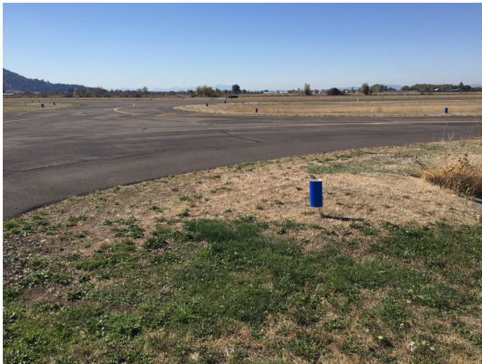
Taxiway reflective-can edge identification
