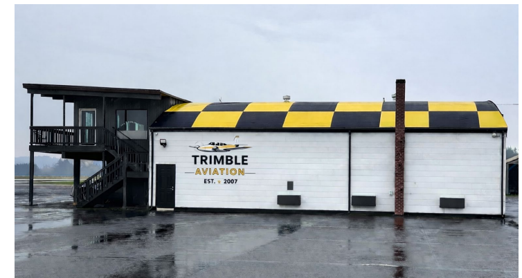
Renovated Quonset hangar
