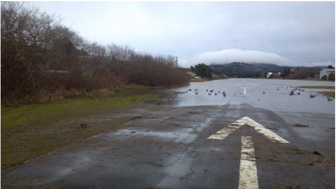
Runway 14 threshold. Facing south.
