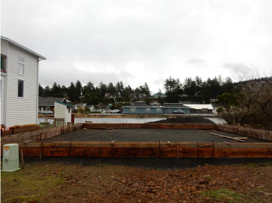
Facing east from Rueppell Ave. Flooded runway in distance.
