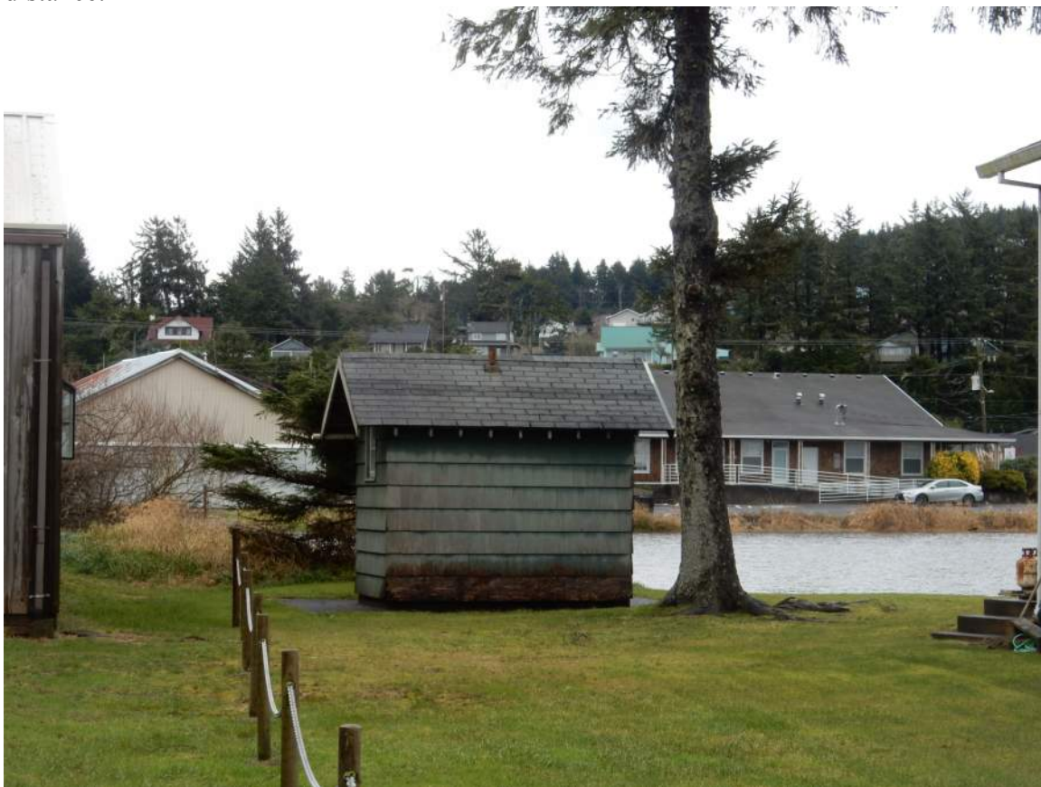
Facing east from Rueppell Ave. Restroom north of tie down area (submerged). Private land in foreground.
