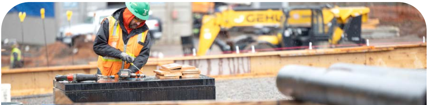
| A contractor working on a jobsite.
