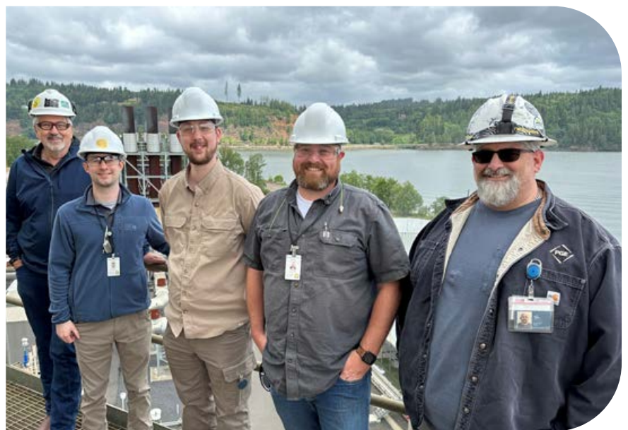
BCD boiler and pressure vessel inspectors – pictured from left, Bob Graham, Tom Clark, Patrick McGiveron, and Jon Everitt – visit the Port Westward power plant in Columbia County to learn about Portland General Electric's heat recovery steam generator. Also pictured, at right, is Chris Baier, chairperson of the Oregon Board of Boiler Rules.
