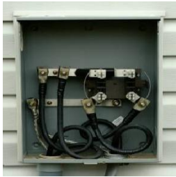
Step 2a Hi-Lug Ground Installation
