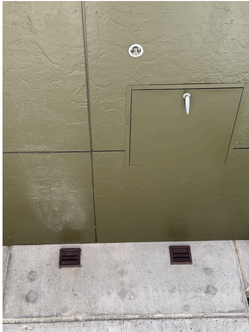
Photo showing a white "rust" located superior to the applicant's kiln exhaust vent (lower left-hand corner of the image).
