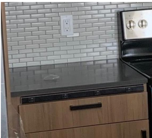
Outlet in front of cabinet where drawer height is reduced
