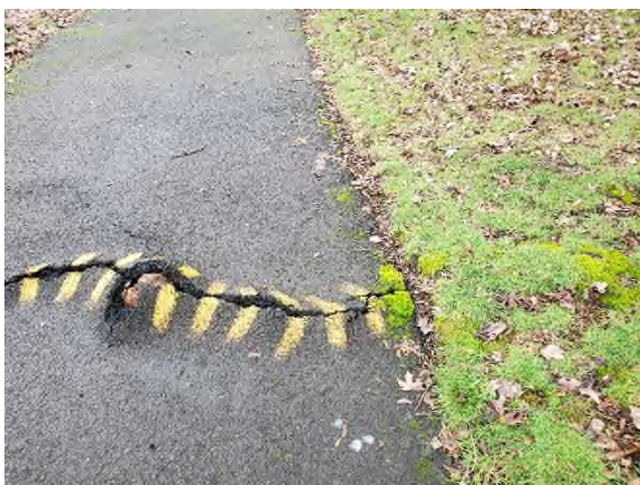
Cracks on paving
